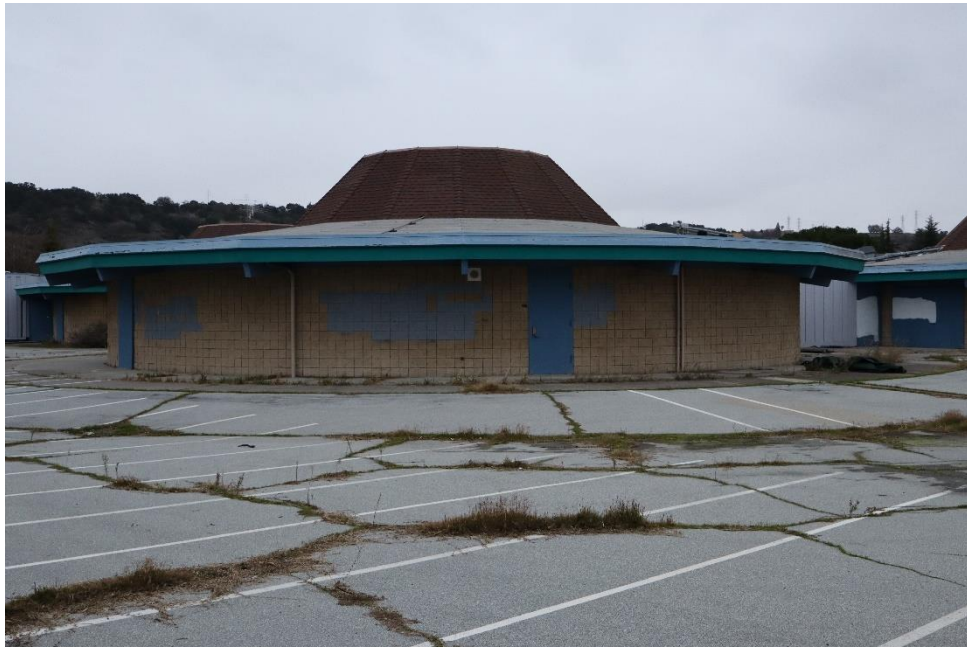
Figure 19. Showing the northeastern-most rotunda, facing south.
