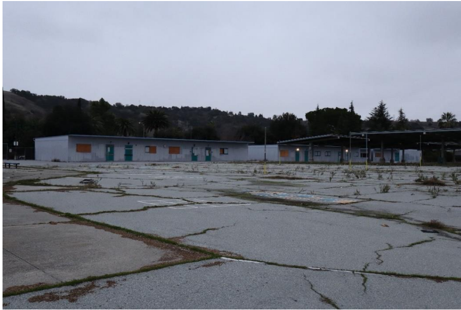
Figure 28. Four portable classroom buildings, facing northwest.
