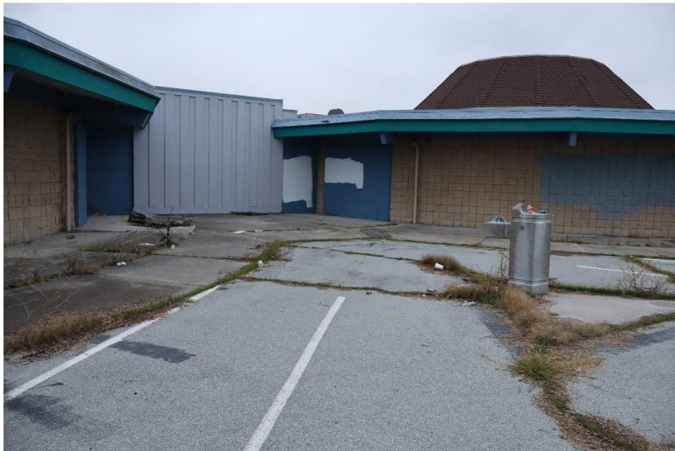
Figure 3. Showing an exterior, integrated wooden wall that joins the two most northerly rotundas, facing southwest.
