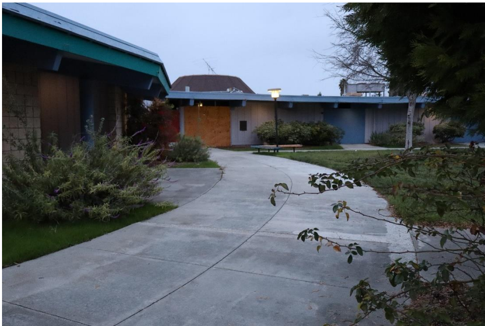
Figure 5. Photograph showing a section of Unit B, adjacent to Unit C, facing east.
