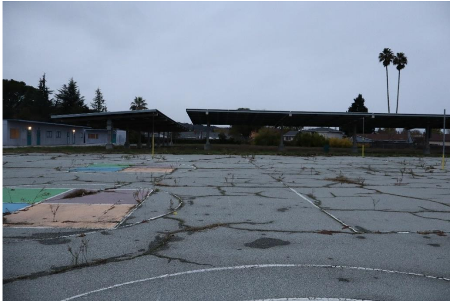
Figure 11. Photograph showing the 2017 solar panels, and a portion of the schoolyard, facing north.
