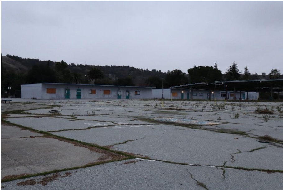
Figure 10. Four portable classroom buildings, facing northwest.
