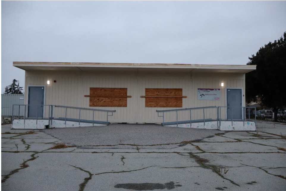
Figure 8. Primary façade, facing east.
