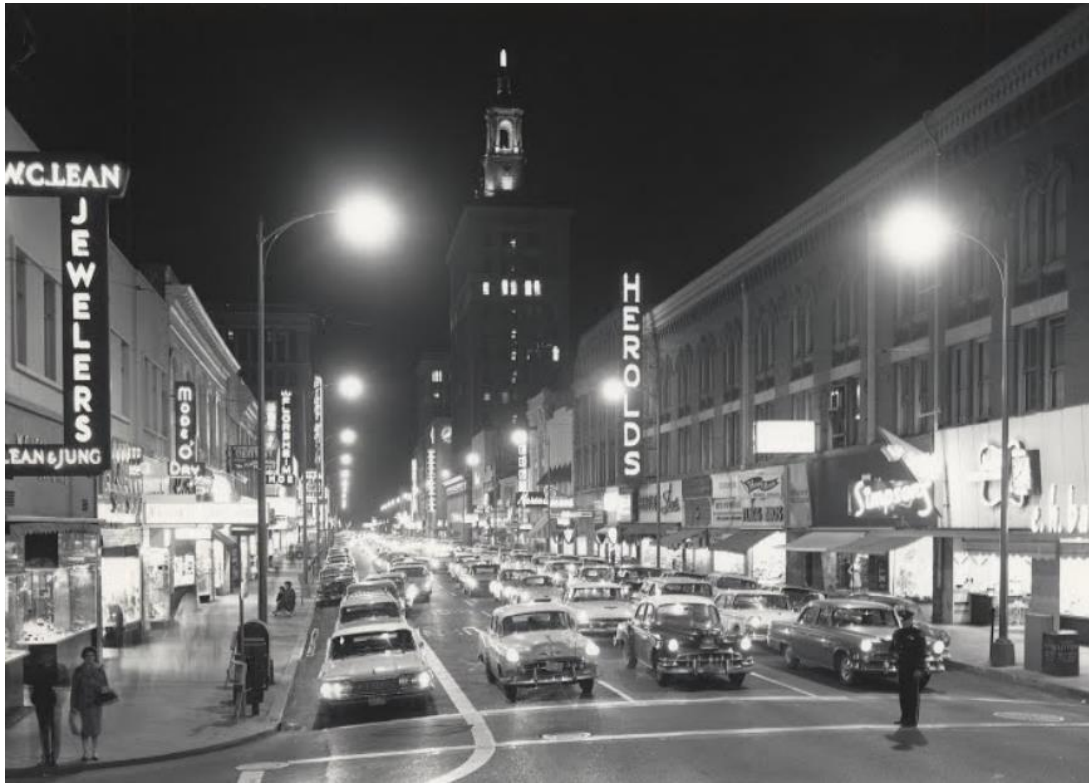
Figure 10. ca. 1955 photograph of S. 1 st and San Fernando streets in downtown San Jose (courtesy of San Jose Public Library, California Room).
