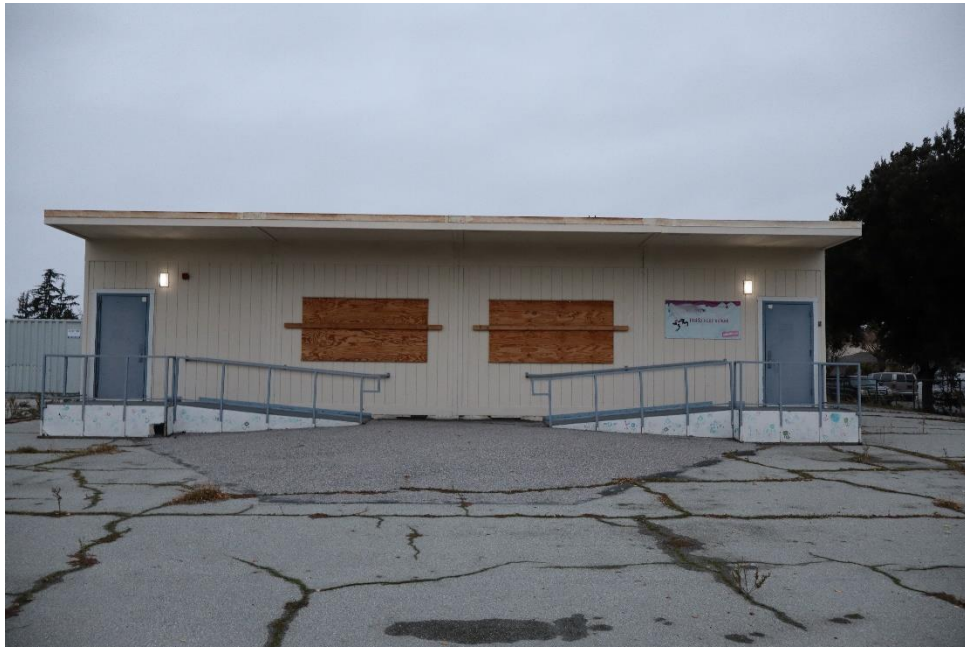
Figure 26. Primary façade, facing east.
