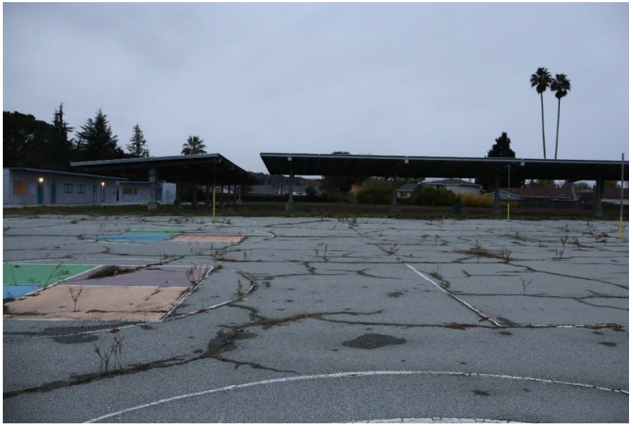
Figure 29. Photograph showing the 2017 solar panels, and a portion of the schoolyard, facing north.
