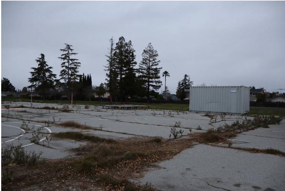
Figure 9. ca. 2002 steel container, facing east.
