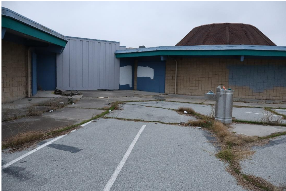
Figure 21. Showing an exterior, integrated wooden wall that joins the two most northerly rotundas, facing southwest.
