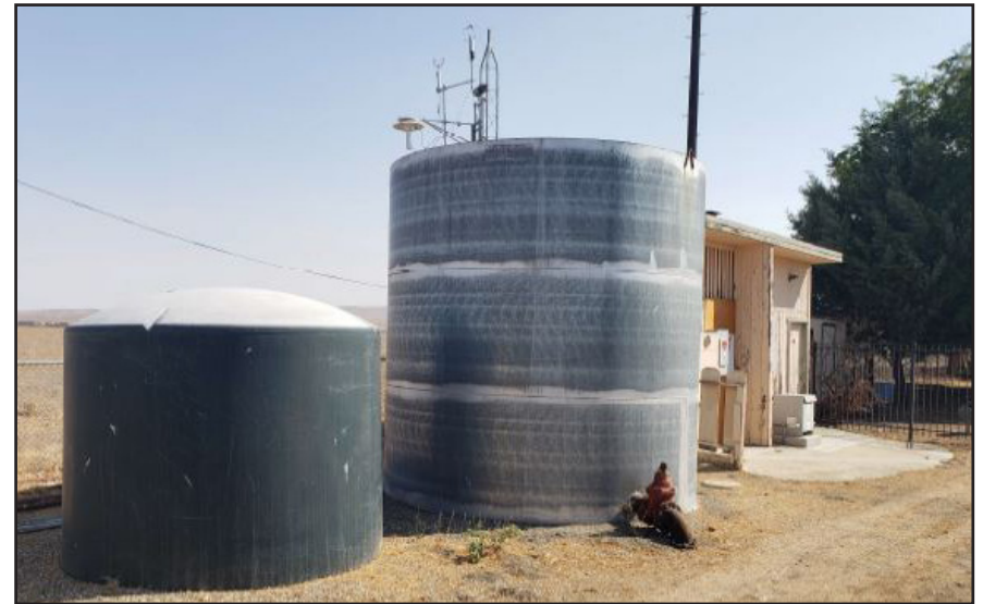
Photo #4: Northeast facing view of storage tanks and well building from project site. (Source: MNS Engineers, 2024)
