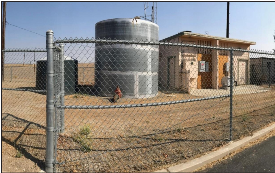
Photo #3: North facing view of storage tanks and well building from project site. (Source: MNS Engineers, 2024)
