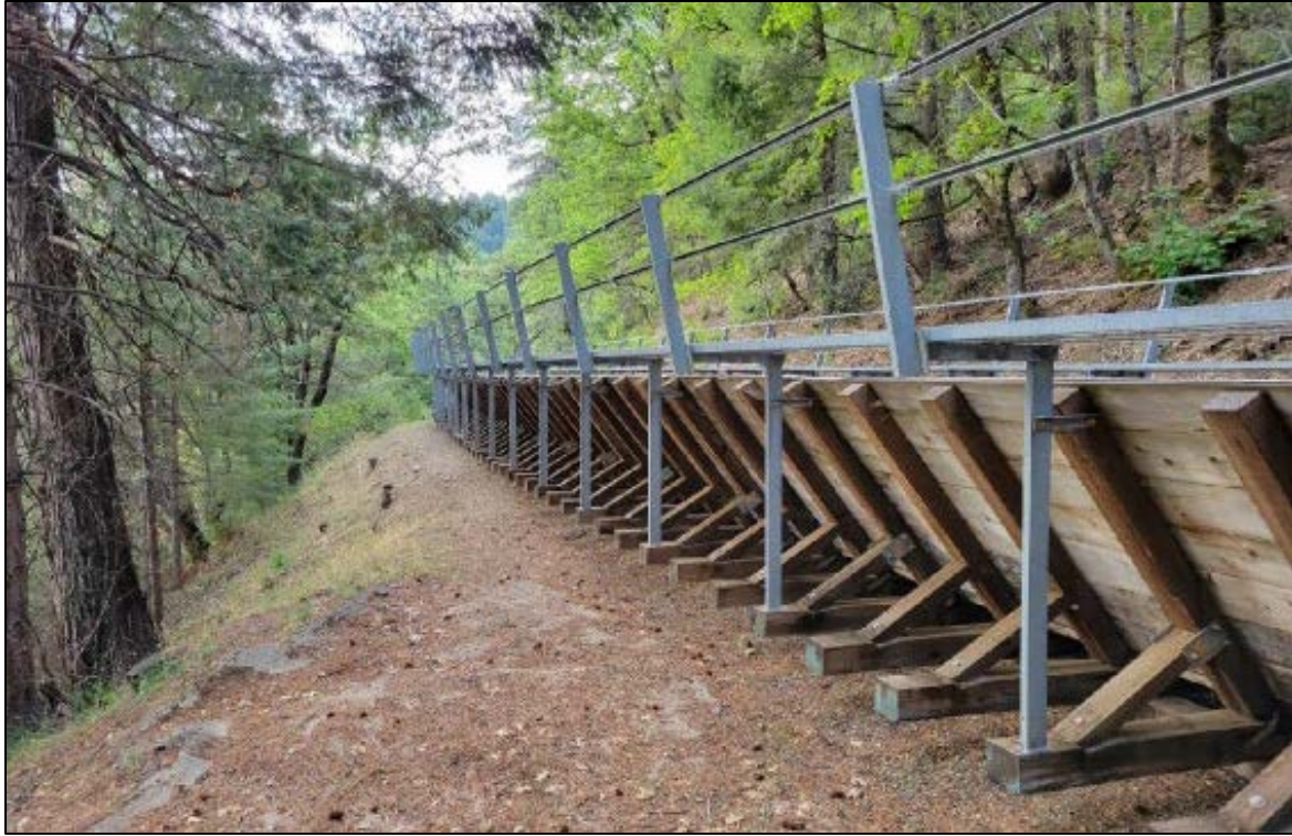
Figure 2.4. Photo of Underside of Flume 45 Wooden Substructure
