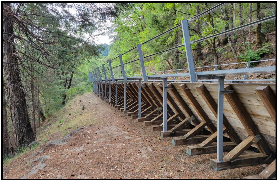
Photo 2: Flume 45 wooden substructure
