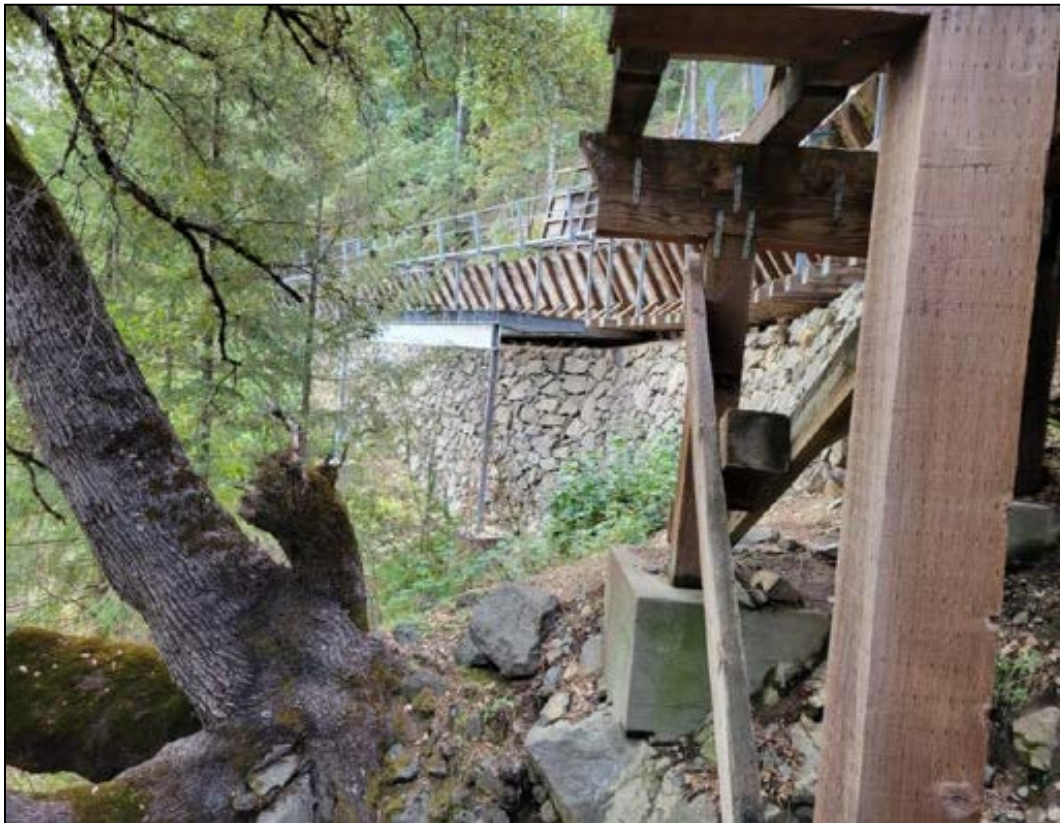
Figure 2.5. Photo of Flume 45 Historic Rock Wall Foundation
