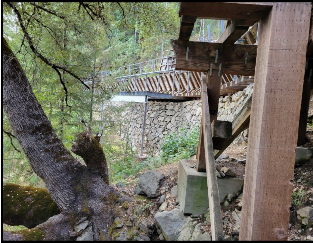
Photo 3: Flume 45 rock wall foundation
