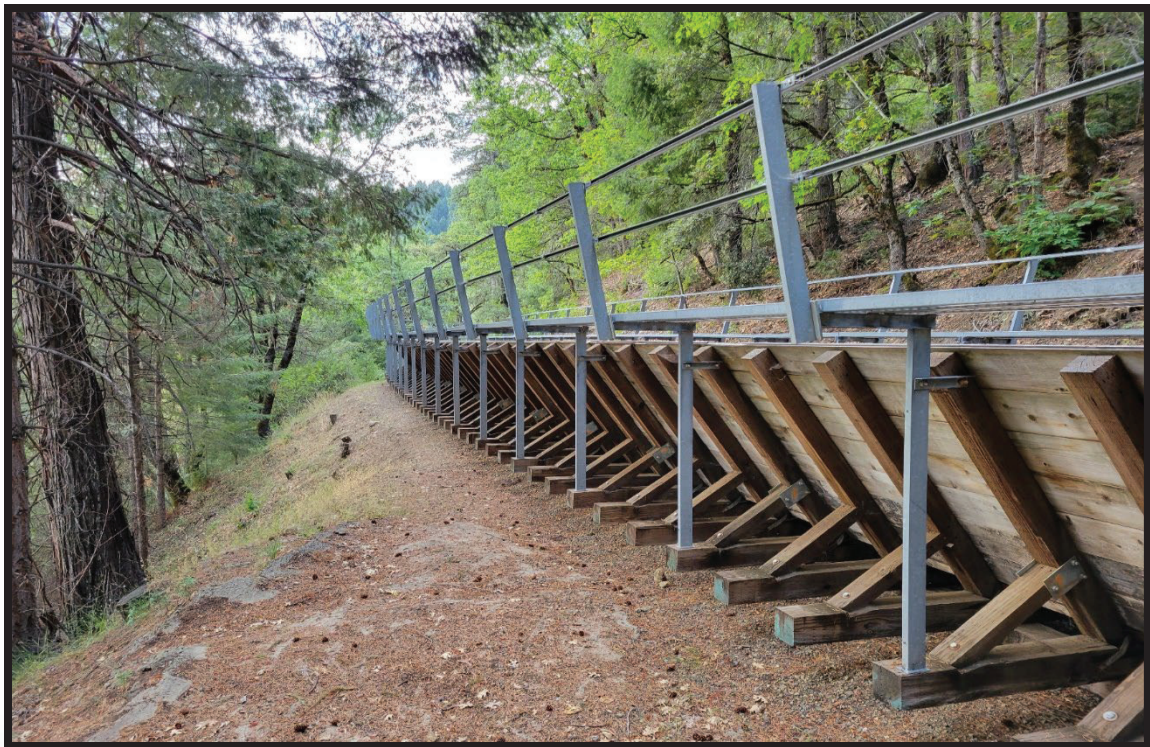
Photo 2: Flume 45 wooden substructure
