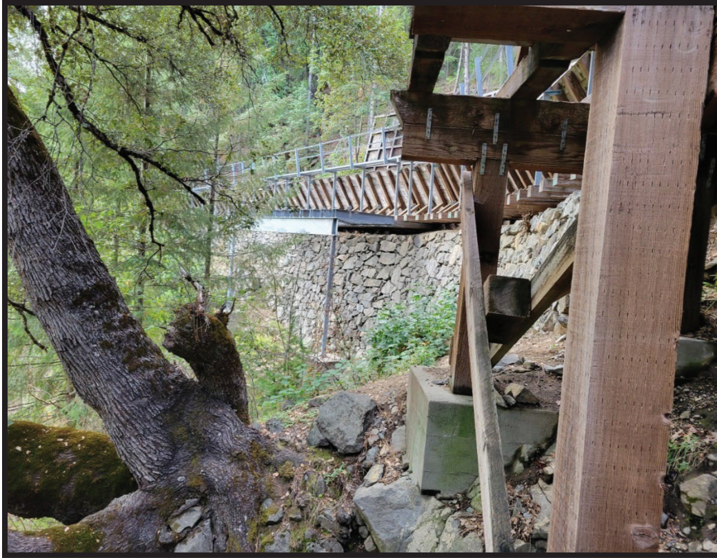
Photo 3: Flume 45 rock wall foundation
