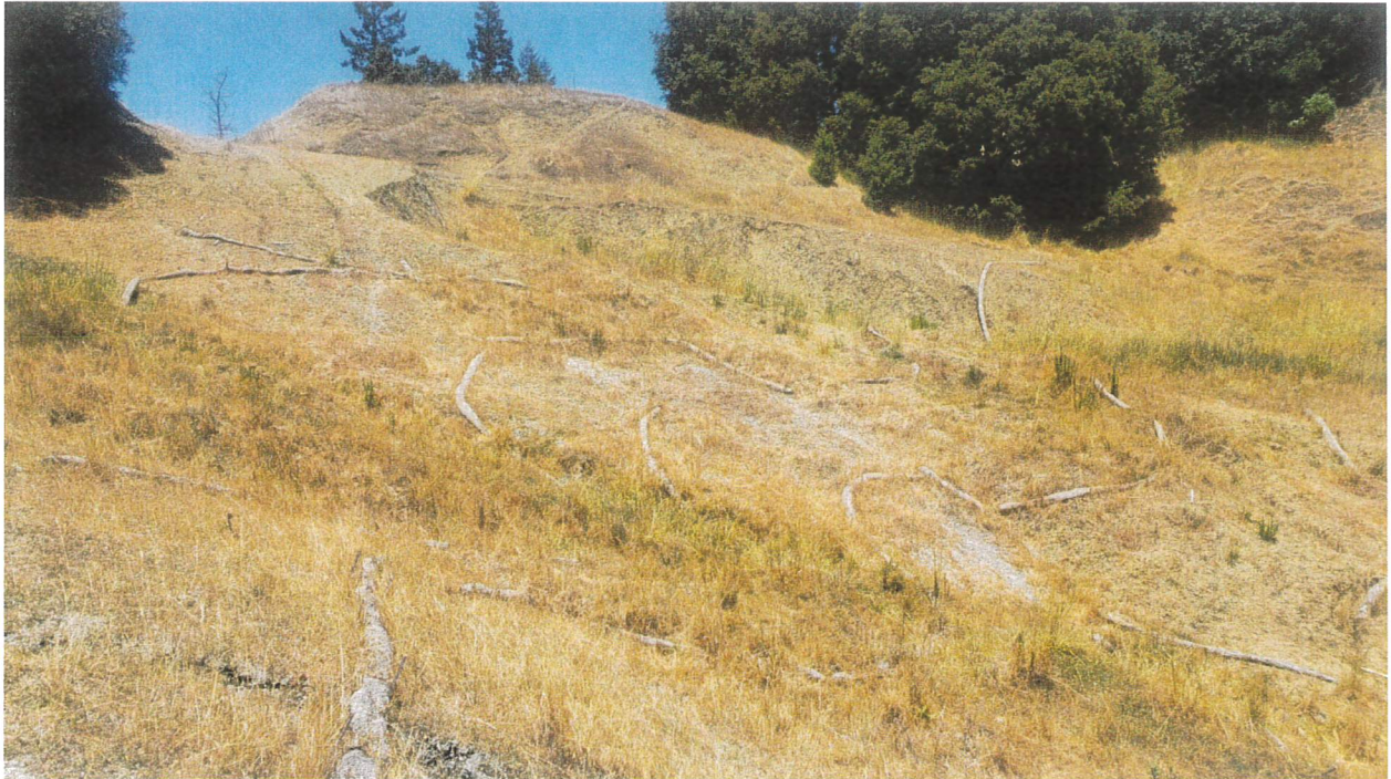
Photograph of the road fillslope failure at Site 36 taken from the west.
