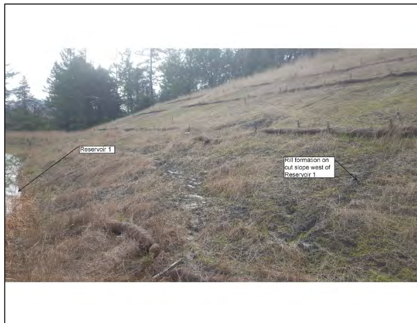
Photograph 4. The cut slope on the west side of Reservoir 1. Rills have formed, but nothing meeting the definition of stream was present.
