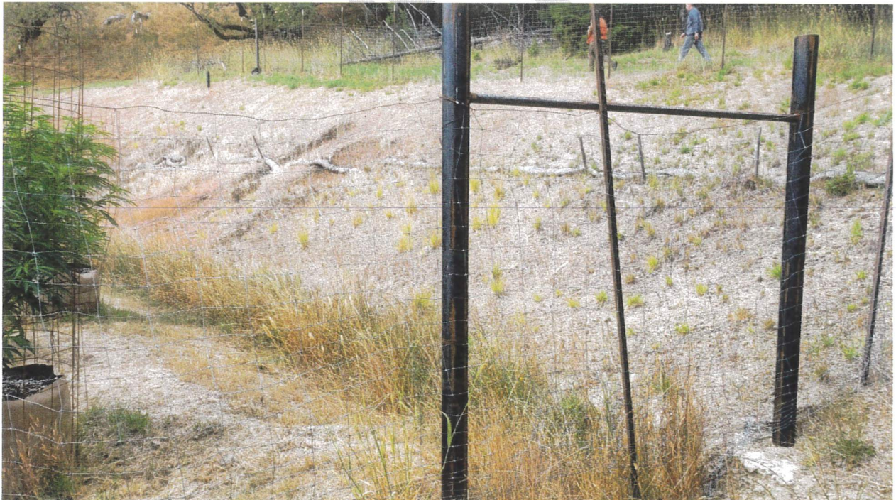
Looking at the drainage ditch along the northeastern side of Cultivation Area A. The diverted watercourse from Site 21 is draining over the cut bank and causing the erosion of the cutbank as scene in this photograph.
