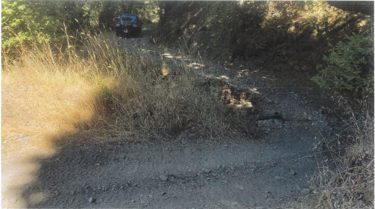
Photograph of the watercourse crossing at Site 16. This crossing is to be upgraded to a culverted crossing and the road approaches rocked to the garden parking area immediately to the left out of frame of this photograph.
