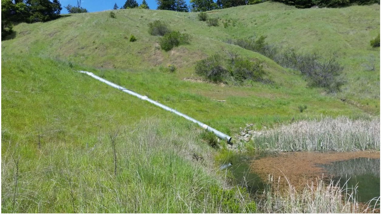
Photo 3. Culvert connected Upper Pond with Lower Pond
