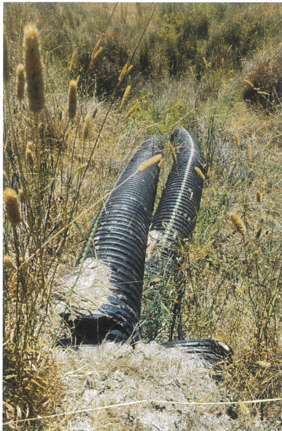
Photograph of the failing secondary spillway at Site 39. This spillway is to become the primary spillway after reconstructing of the pond embankment and installation of an anchored 24" culvert spillway.
