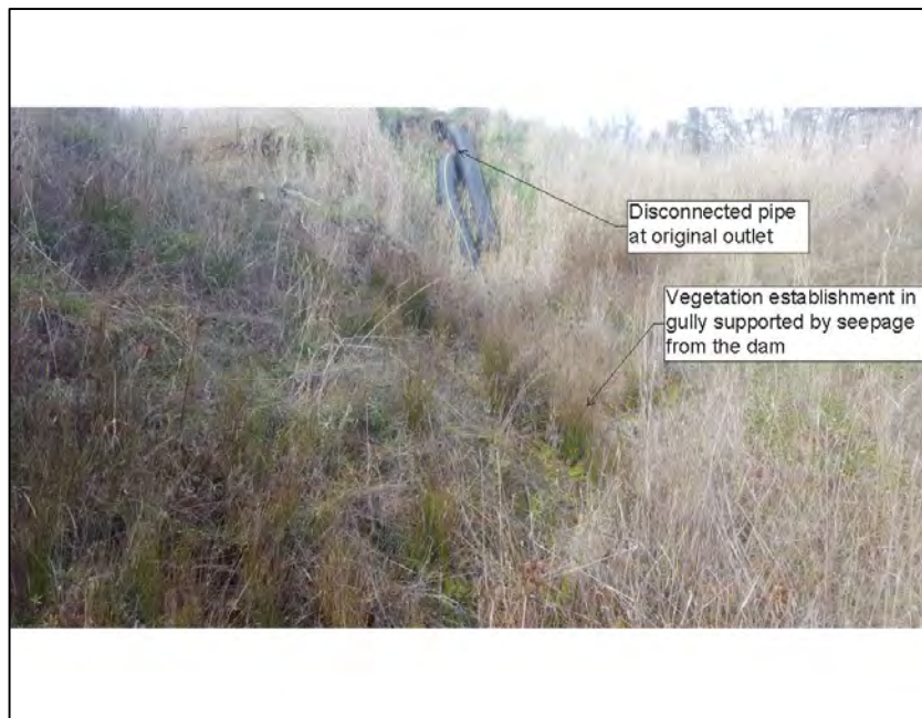
Photograph 6. Gully below Reservoir 2 eroded by outfall from the reservoir from the drain pipe separating. A new outlet on the east side of the reservoir was installed. Seepage from the bottom of the reservoir is becoming established
