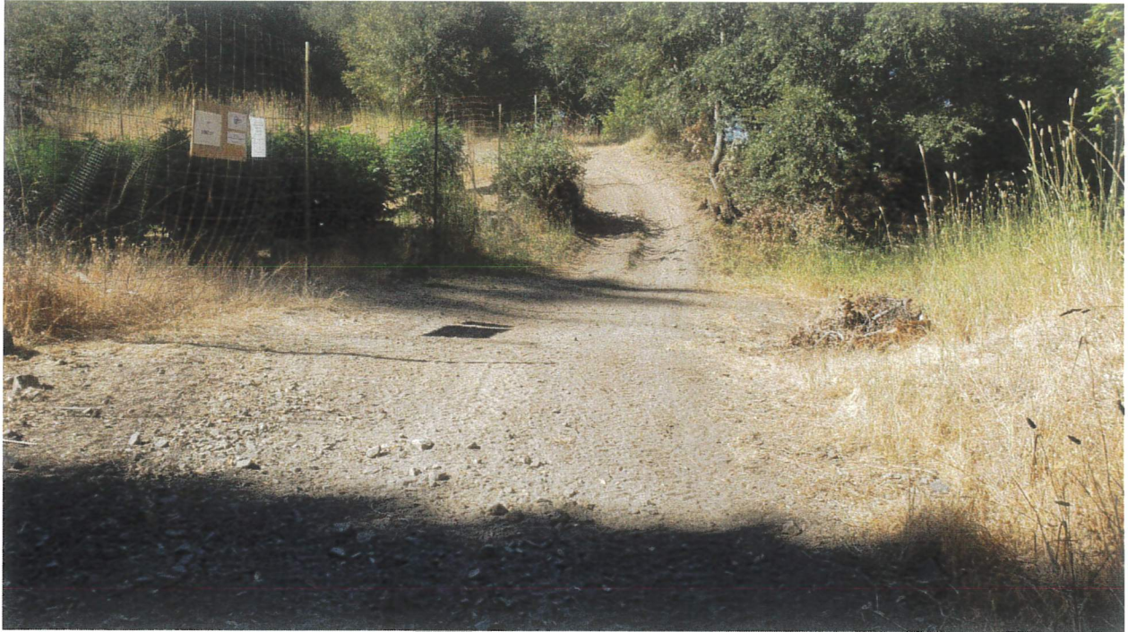
Photograph of Cultivation Area B's parking area. This area is to be rocked and staked straw wattles are to be installed to the right of the road along the brush line above the watercourse.
