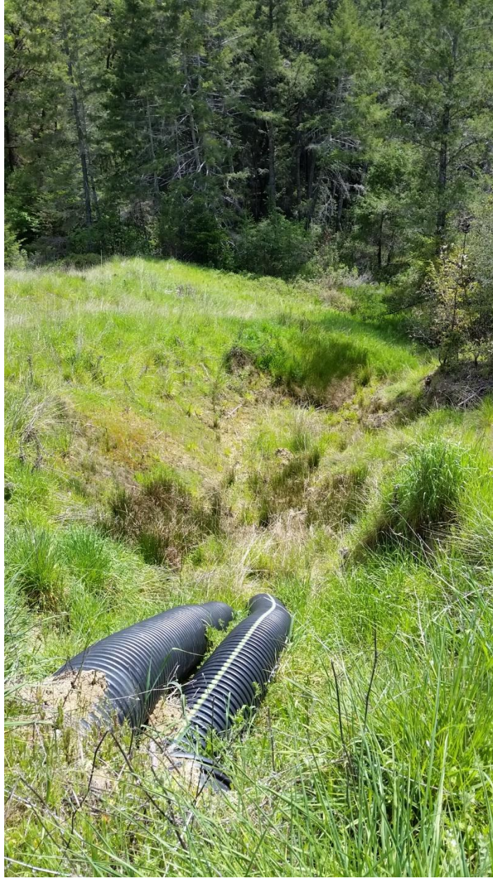
Photo 5. View of culverts behind earth dam of Lower Pond and erosion, with Class II drainage below
