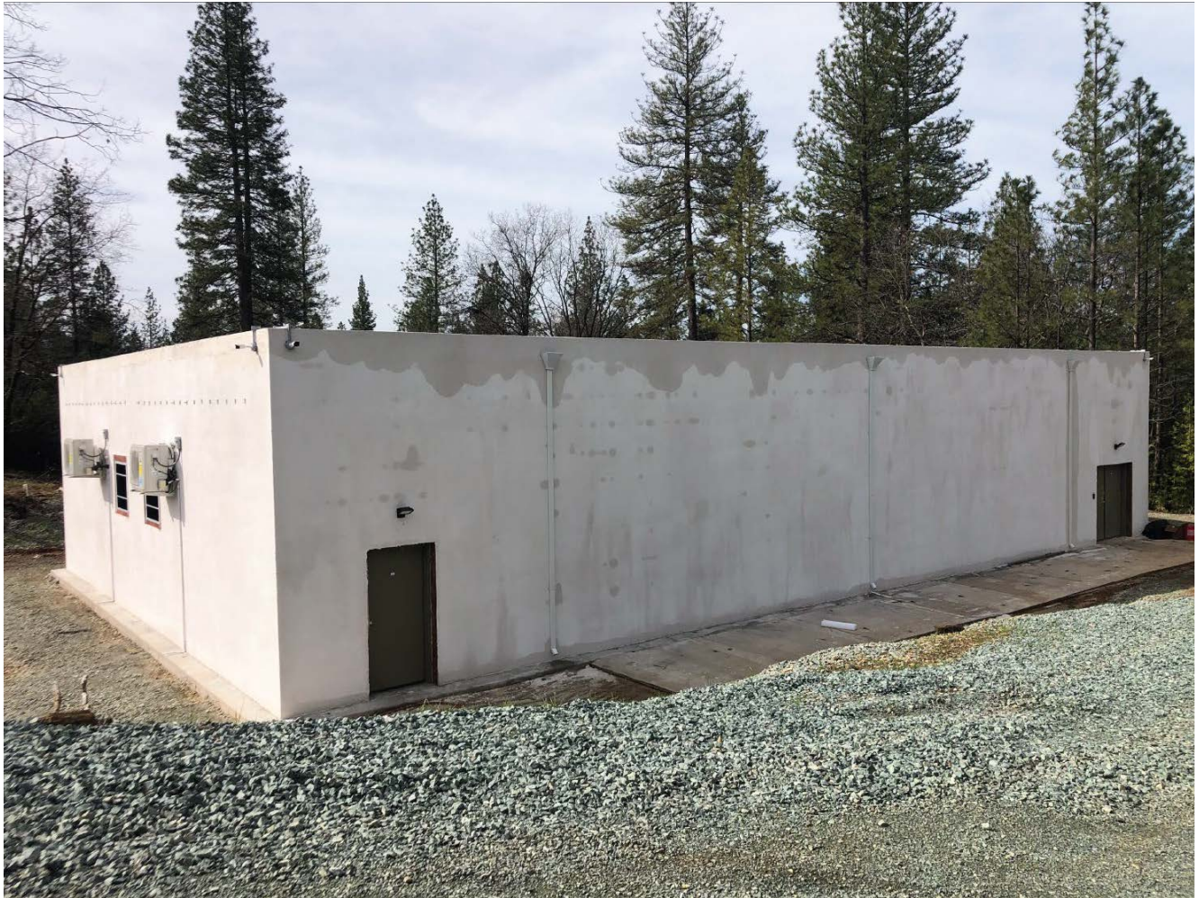
Figure 4: Drying Building, Photo via Pinecrest Research Corporation, Inc.
