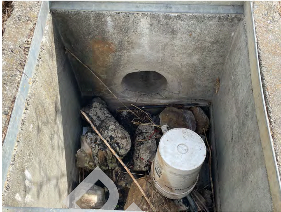
23. Detailed view of hole feature; appears to be an unused stormwater drain
