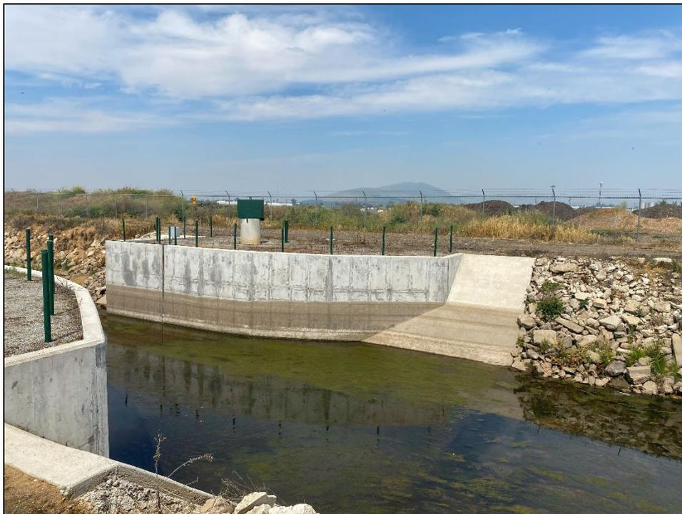
**Figure 9.** Wutchumna Canal/Ditch overview showing concrete walls and ramp leading down into ditch, 2024. Large riprap installed on soil slope of ditch to control erosion. View toward northwest.
