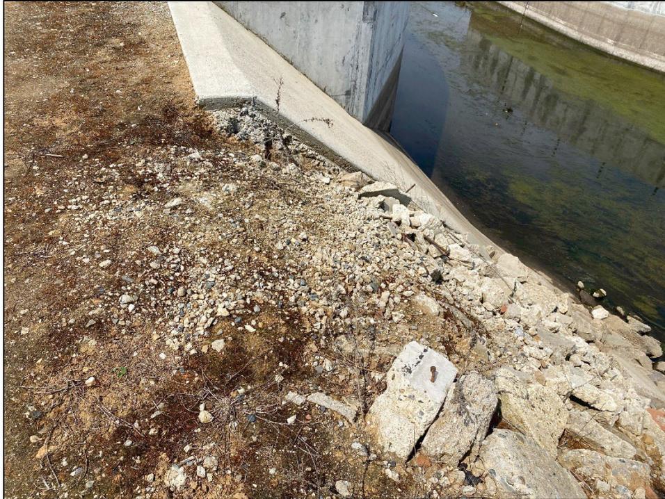
**Figure 8.** Detail of riprap and rubble placed adjacent to concrete ramp on south side of Wutchumna Canal/Ditch, 2024. View toward west.
