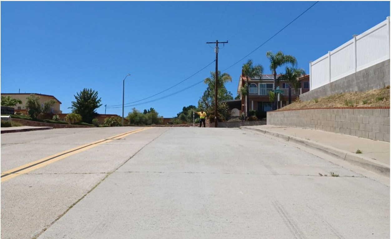
Figure 14 - Stopping Sight Distance Traveling Northbound Towards Project Driveway #2 = 113'
