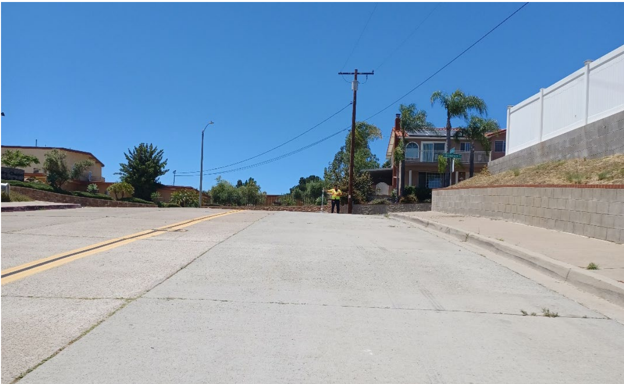
Figure 10 - Stopping Sight Distance Traveling Northbound Towards Project Driveway #1 = 115'
