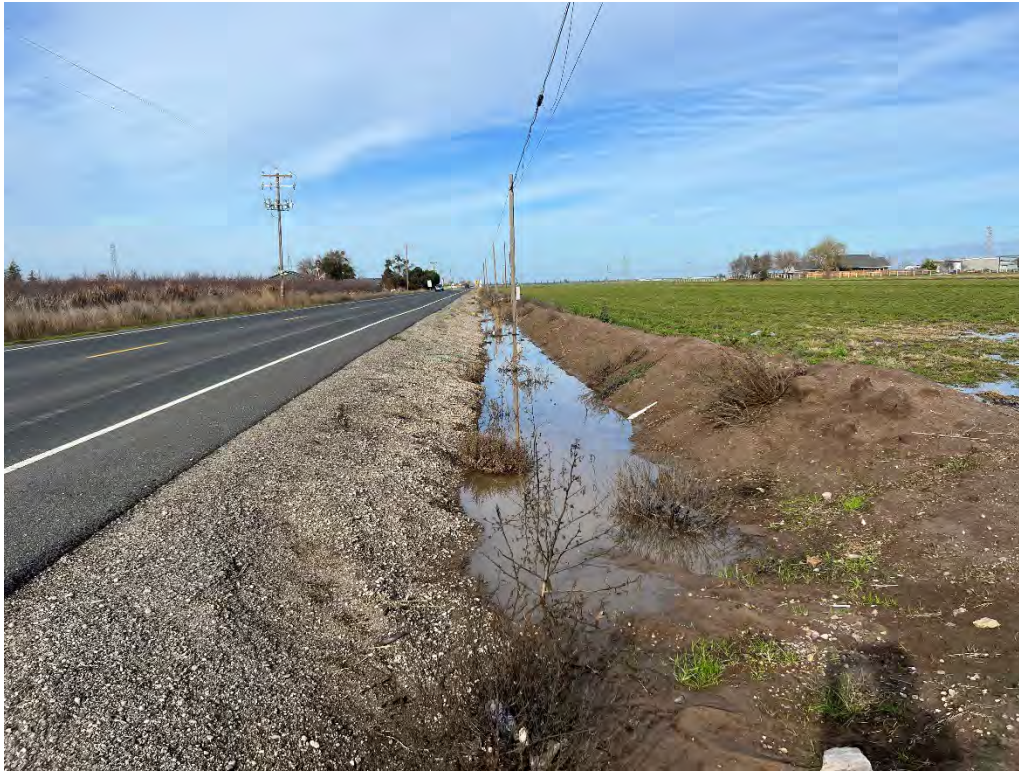
Photograph 43: From the eastern shoulder of Escalon-Bellota Road, looking north through an existing roadside ditch.
