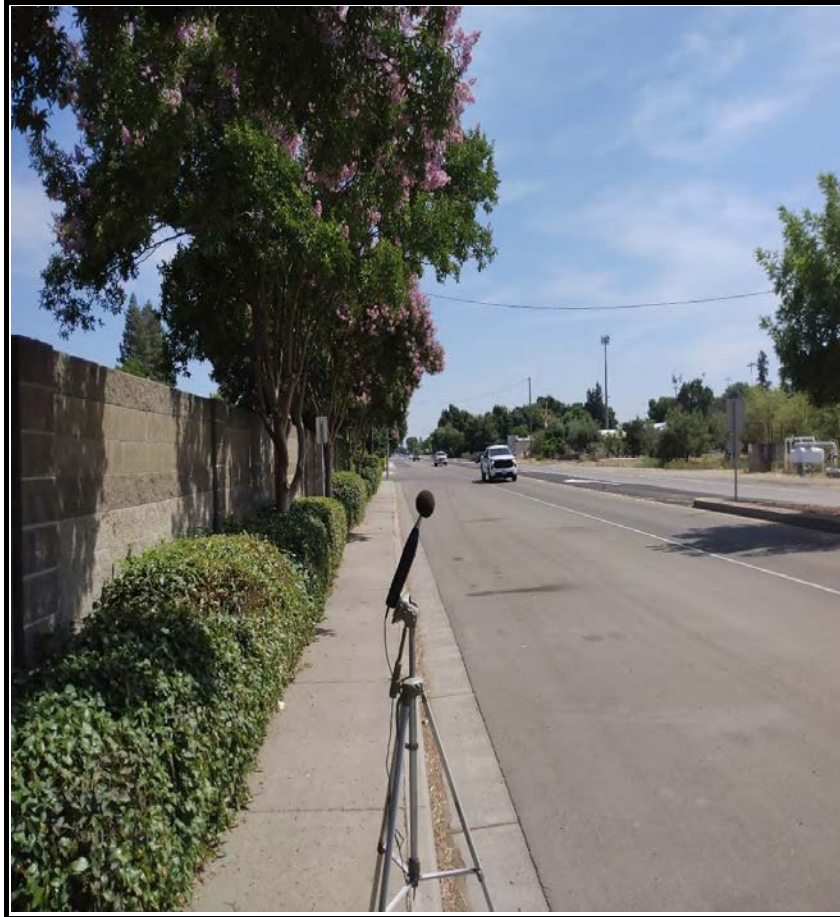
STNM4 looking S down Escalon- Bolleta Road. Backyard to residence 209 Tiffany Ct on other side of ~7' tall block wall (left of image). Feed store building, 17407 Bellota Rd, ~600' SSW (on right of image across the road).
