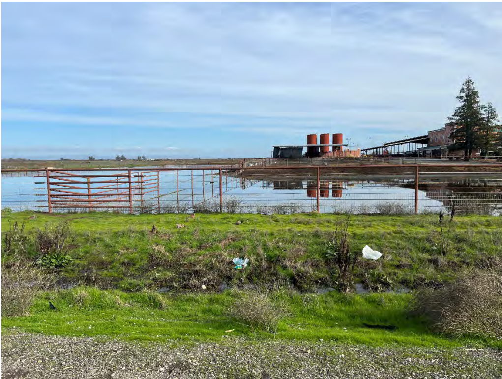
Photograph 28: From the eastern shoulder of Escalon-Bellota Road, looking east at existing roadside ditches.
