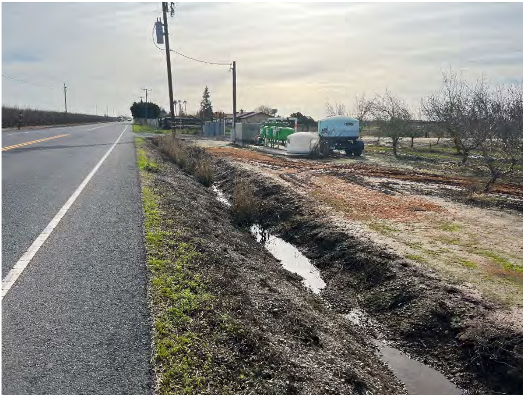
Photograph 30: From the intersection of Escalon-Bellota Road and Edwards Avenue, looking south along Escalon-Bellota Road at existing pumps and tanks adjacent to a roadside ditch within the project site.
