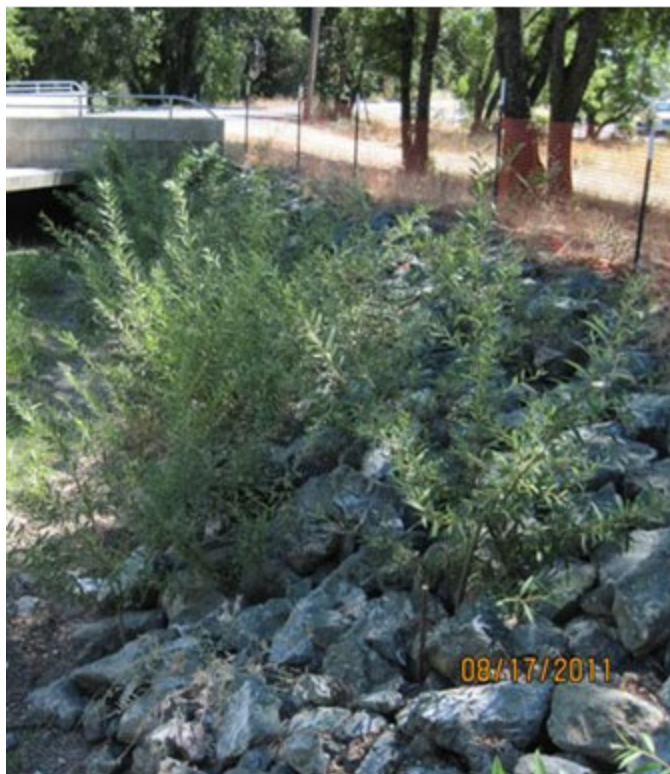
Figure 18- Gibson Creek, Cuttings through RSP (Summer 2011)
