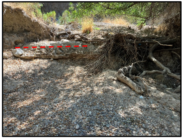
Photo 2. Franklin Creek exposed sewer line, August 7, 2024, view upstream (southwest).
