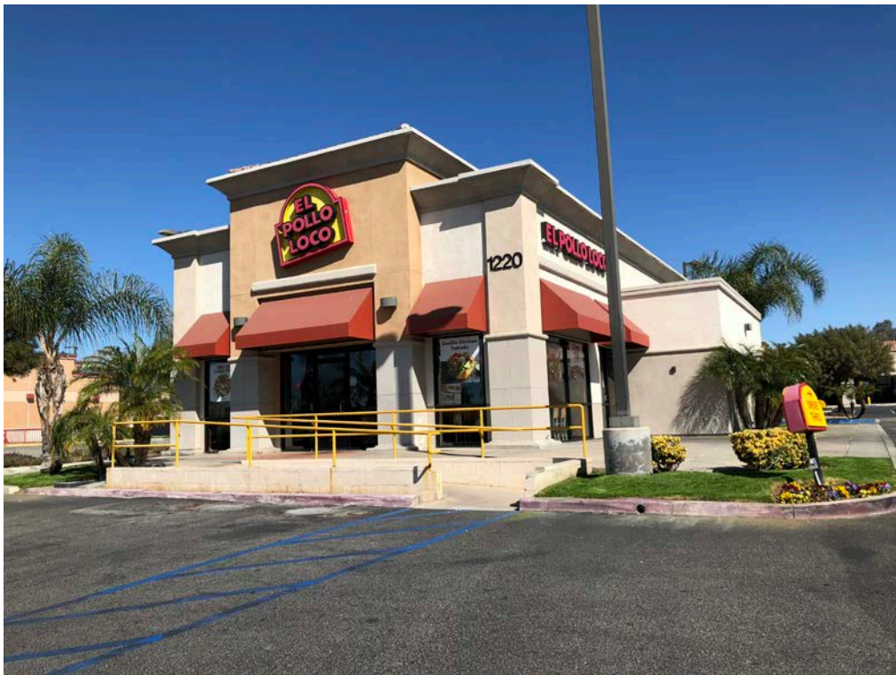
Photo 12: View of adjoining property to the east.
