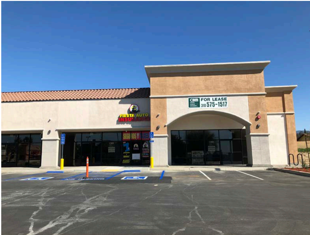
Photo 11: View of adjoining property to the northwest.
