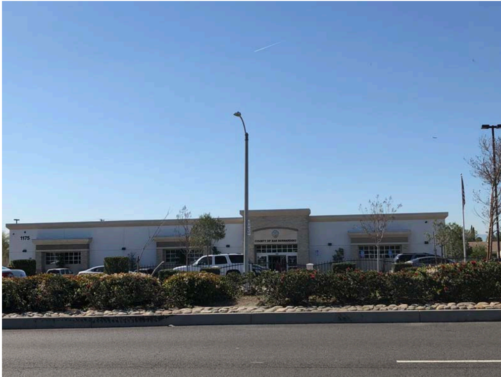
Photo 13: View of adjoining property to the south.
