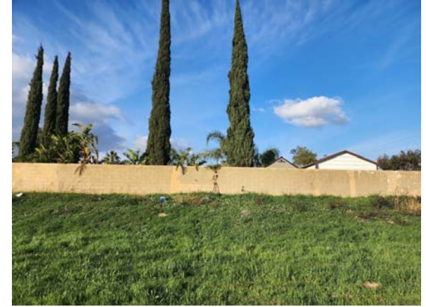
Figure 3: ST-3 140 ft from Larch Ave
