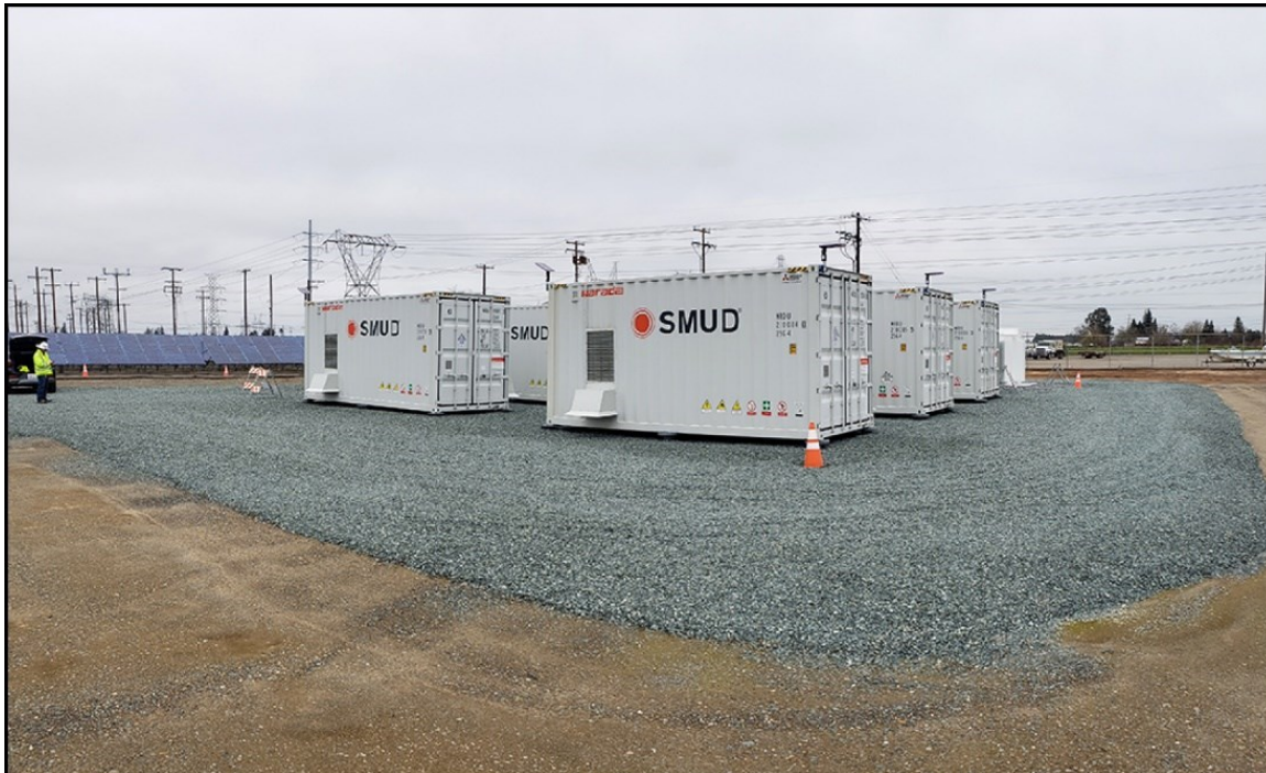
Exhibit 2-9. Battery Energy Storage System
