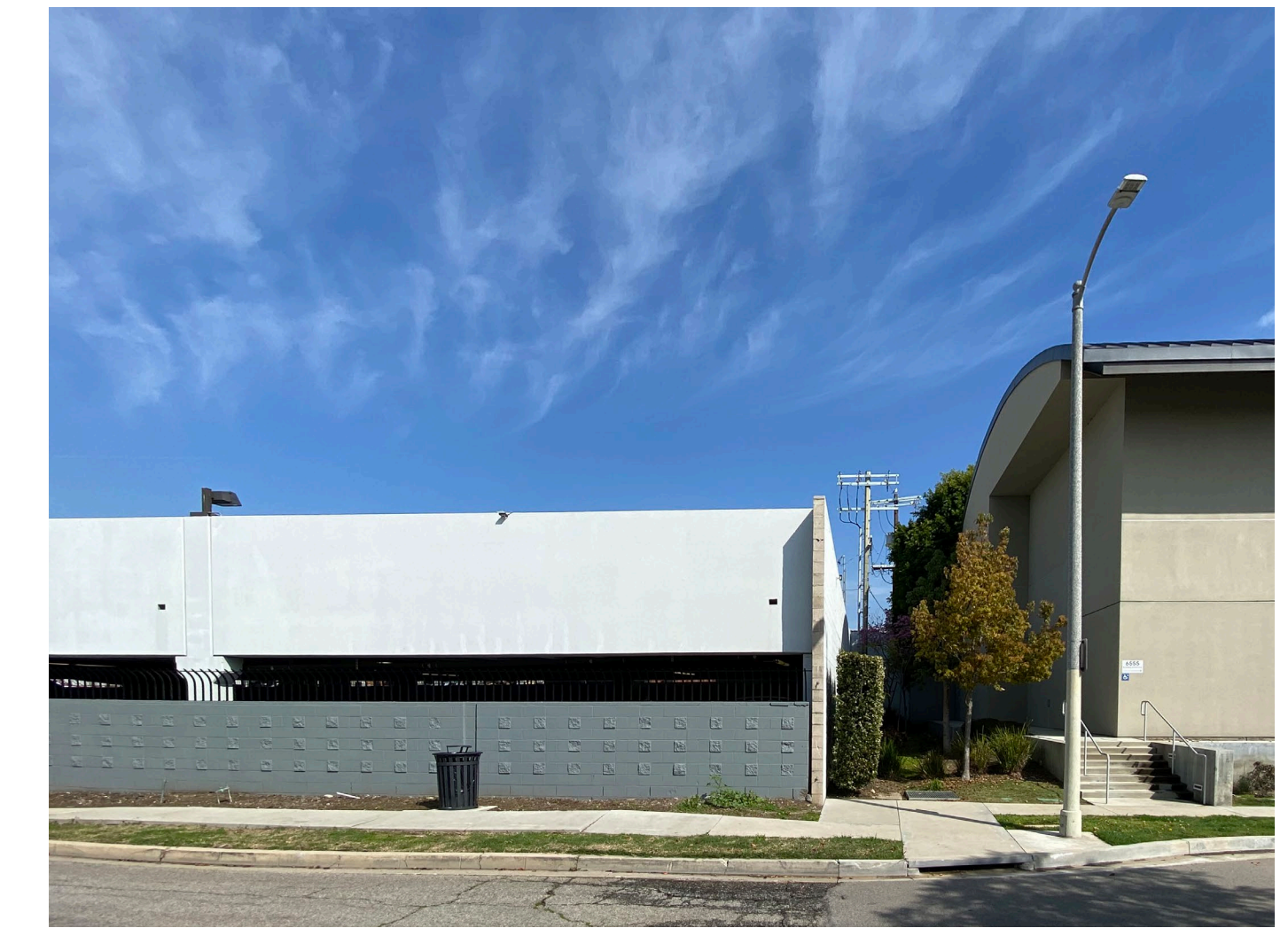
View 6 ▪ Parking garage wall setback from property line
