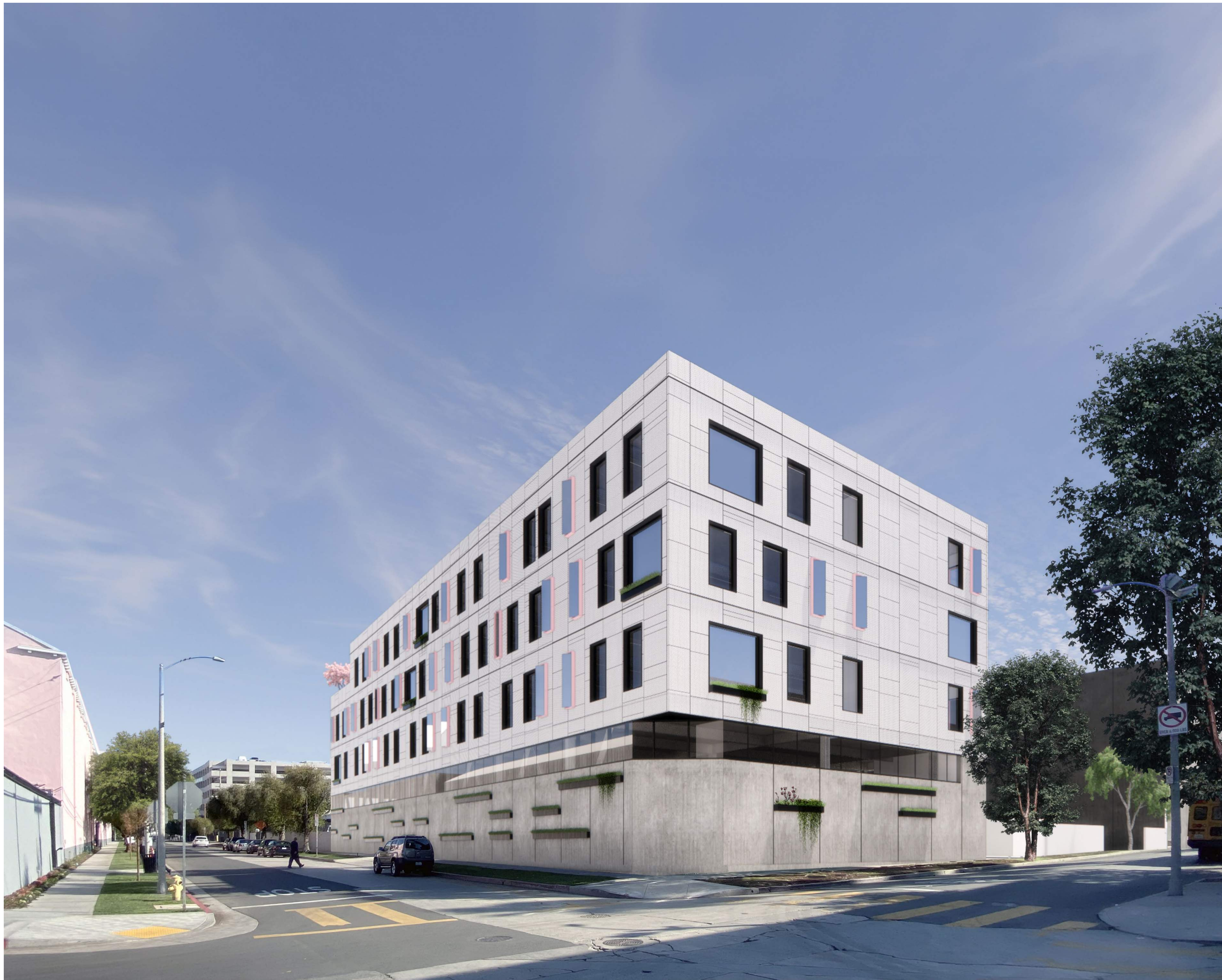
VIEW HEADING EAST ALONG ROMAINE ST
