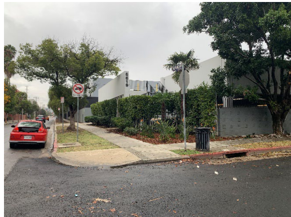
Parking Structure (Figure 2 #3) Looking northeast from Barton Ave.
