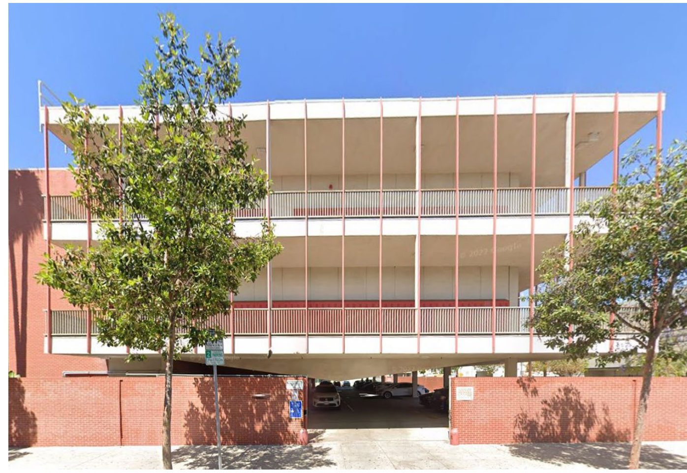
View 1 ▪ Existing middle school on Las Palmas
