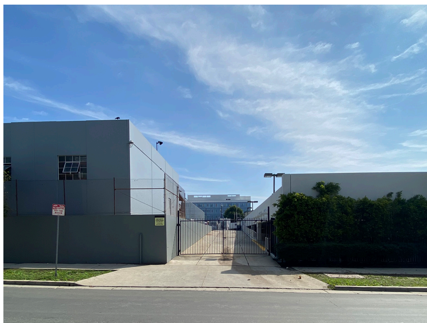
View 4 ▪ Existing curb cut at gate on Las Palmas Ave.
