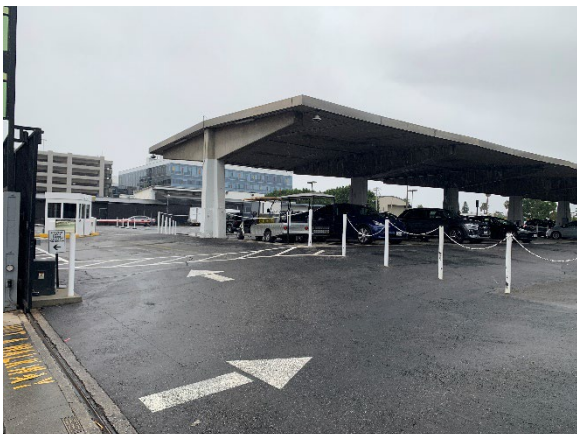
Concrete Canopy/Shed (Figure 2 #4) Looking southeast from Romaine St.
