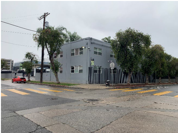
Two-story office building (Figure 2 #1) Looking southeast from the intersection of Romaine St. and Las Palmas Ave.
