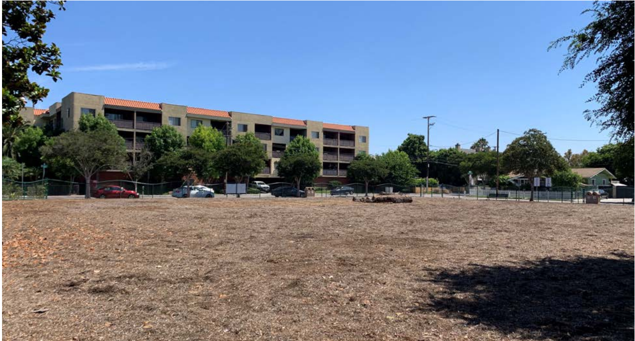
Photograph No. 2: Current site conditions facing northeast.
