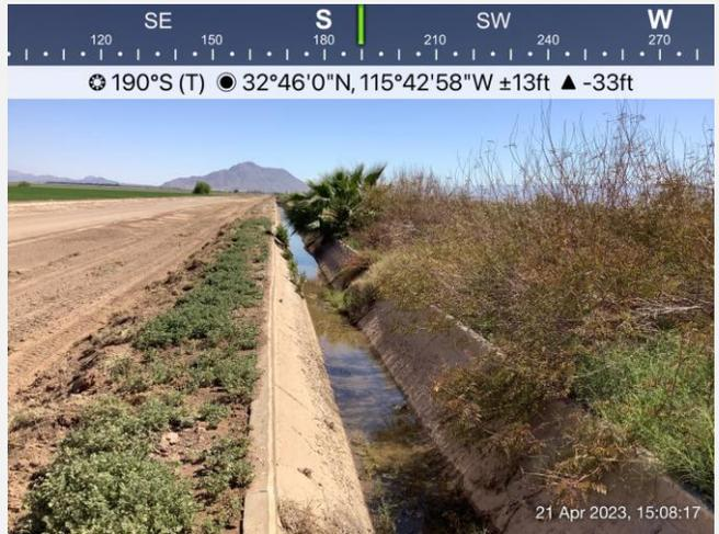
**Photo Point 8:** View of a typical concrete irrigation ditch running north/south that delivers water to smaller isolated ditches.
