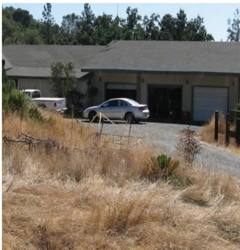
DEFENSIBLE SPACE NONCOMPLIANT
