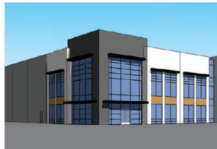
5 BLDG 3 PRIMARY ENTRY
