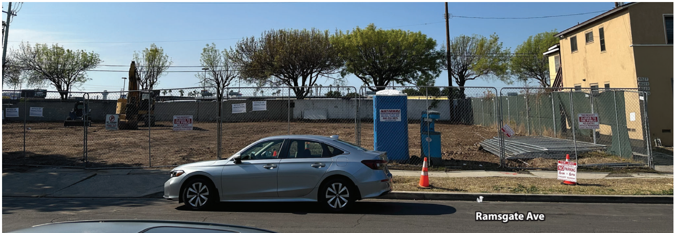
Photo 10 (From E of Project Site Looking W at the E Portion of the Project Site)
