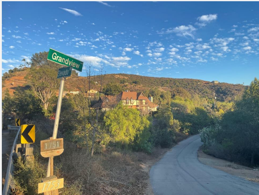
Photograph 19: Photograph taken from Grandview and Elevado Road looking south at intermix homes. Proximity to shrublands and dense residential vegetation increase wildfire risk in this area. Structural ignition risks are exacerbated by wooden home construction materials as pictured.
