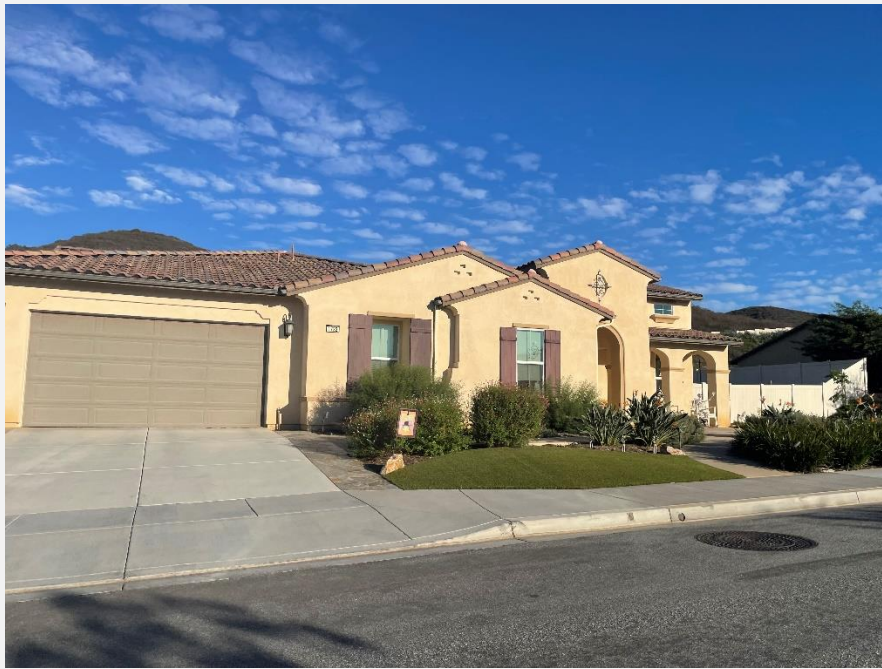
Photograph 11: Newly constructed home on Lemonadeberry Lane showing Chapter 7A construction methods. Structural ignitability could be further reduced by removing the flammable landscaped vegetation directly adjacent to the home.
