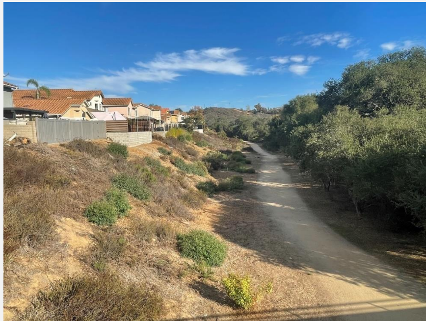
Photograph 5: Photograph taken near the intersection of Green Oak Road and South Melrose Drive looking east at the Fuel Modification Zone of a Wildland Urban Interface community identified as high risk. Vegetation is undermaintained and capable of facilitating wildfire spread.
