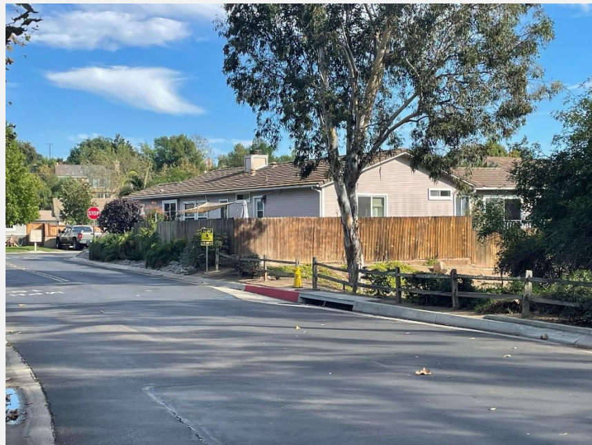
Photograph 14: Photograph taken from Cottontail Drive showing a home adjacent to open space with high load shrubs and chaparral. Wood siding and attached wood fence increase the potential for structural ignitions during a wildfire.
