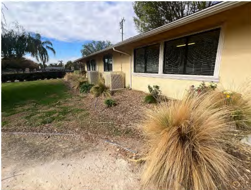
Photo 6: View of the housing units located on the western portion of the Project Site.
