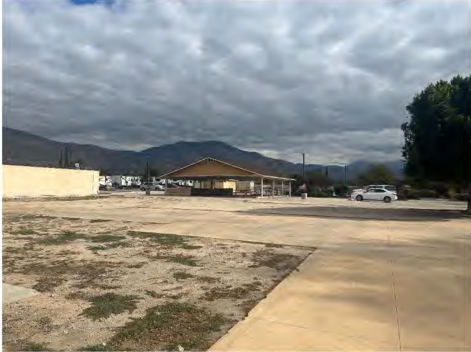
Photo 1: View of existing buildings from the western boundary of the Project Site looking southeast.
