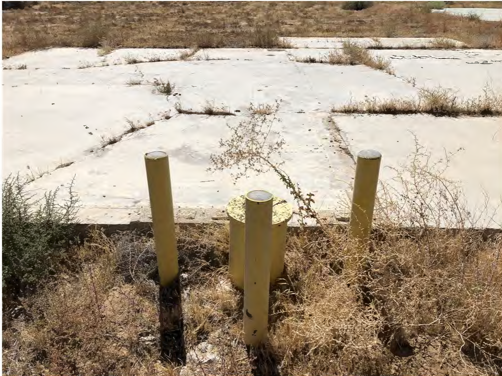
Photo 18 Southern-facing view of northern-most concrete pad. The yellow bollard pictured in the foreground is a marker for subsurface Southern California gas utilities.
