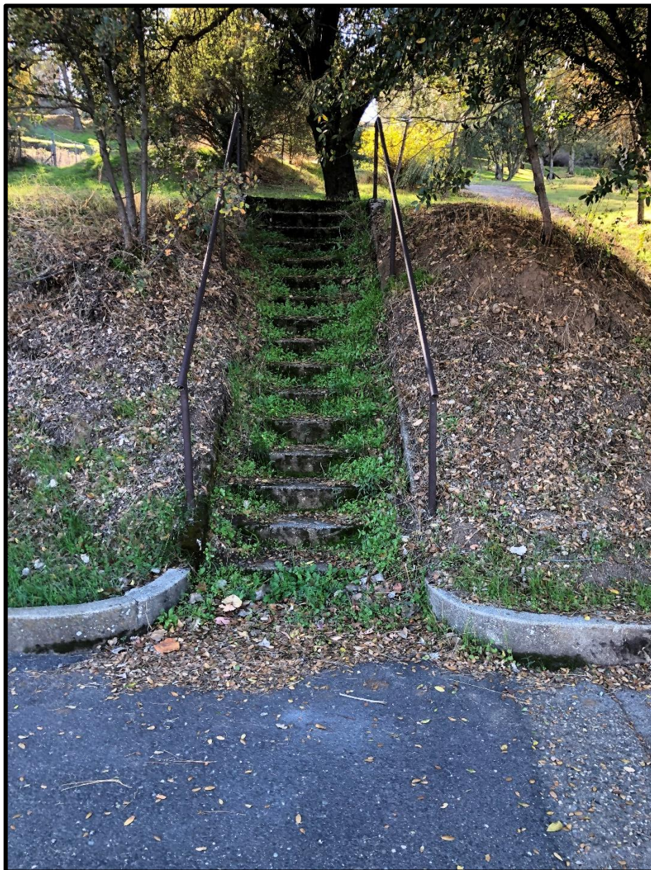
Figure 4.3-7 NULAND RESIDENCE STAIRS FROM EAST ST. CHARLES STREET SIDEWALK; VIEW TO THE SOUTHWEST
