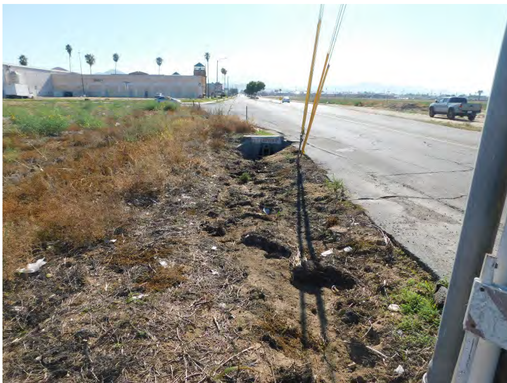
Photograph 11: Looking east toward a culvert which conveys flows under Barrett Avenue to the east of the project site.
