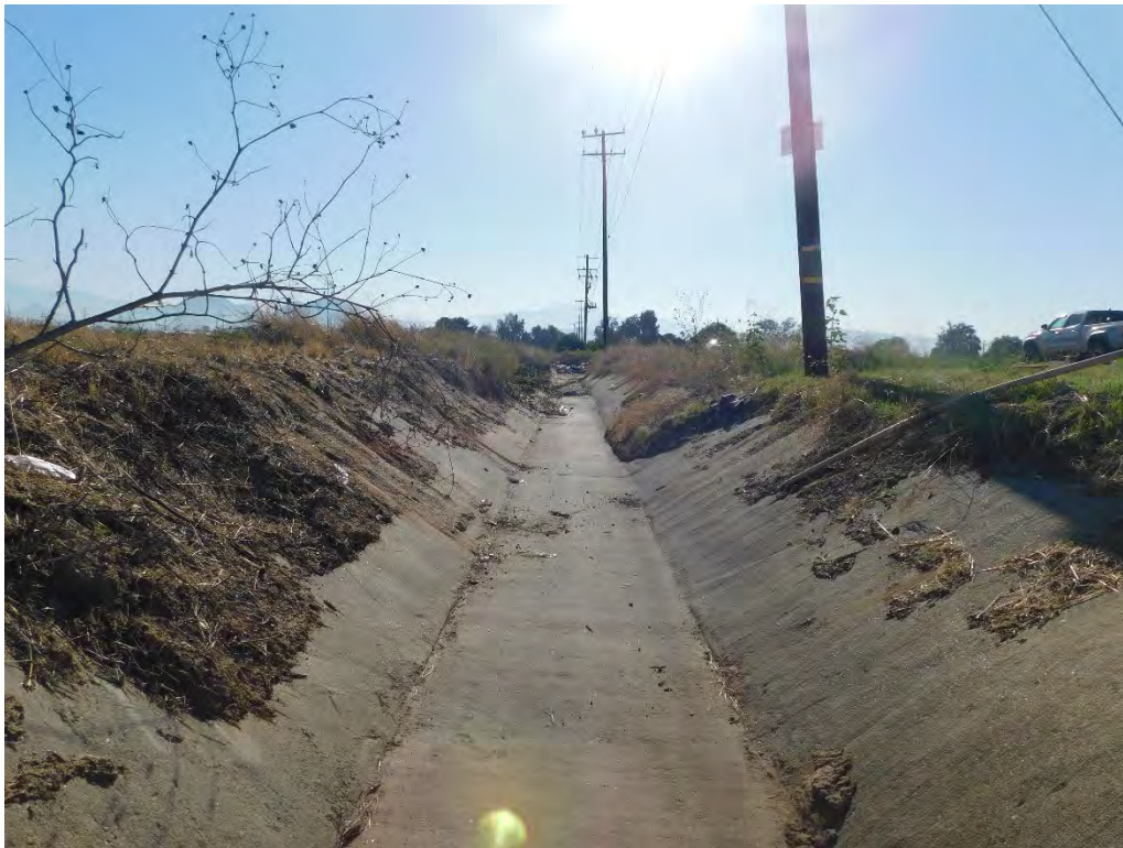
Photograph 7: From the culvert, looking east at the paved portion of the road-side ditch that conveys flows to the east.
