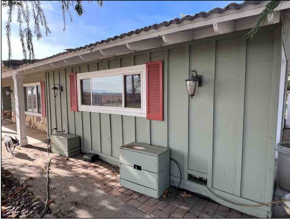
Photo 44. View of the front elevation of the residence, showing the vertical board siding.
