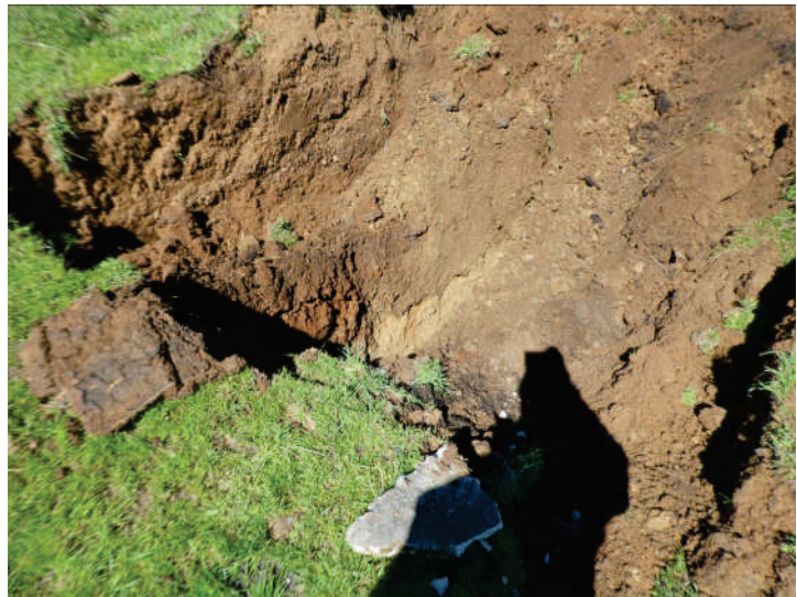
Photo #29: Western soil piles Trench T-9 - Bottom of excavation (5 feet) native soils
