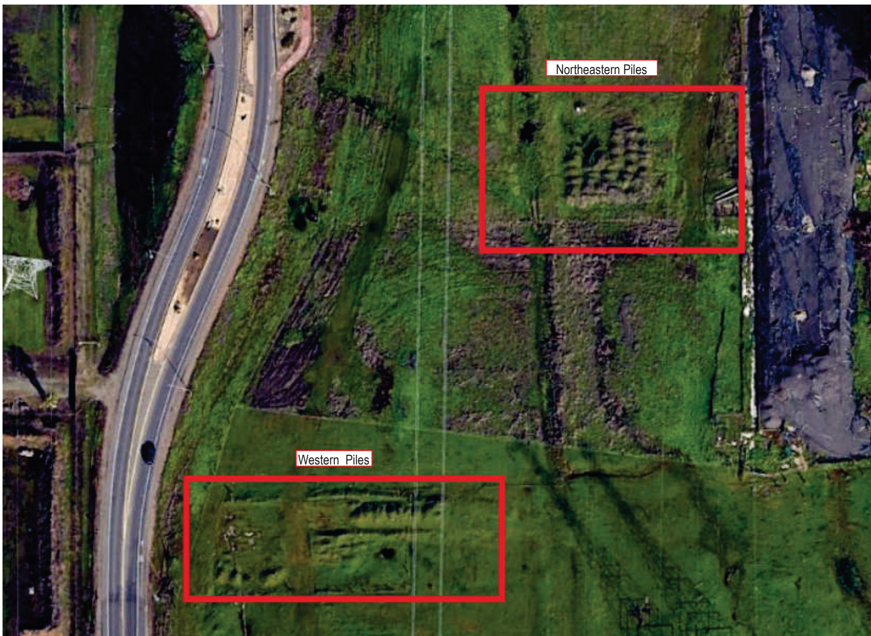
Soil Piles Identified by Geocon/City of Elk Grove Summer Villas – 9350 Sheldon Road, Elk Grove, CA
