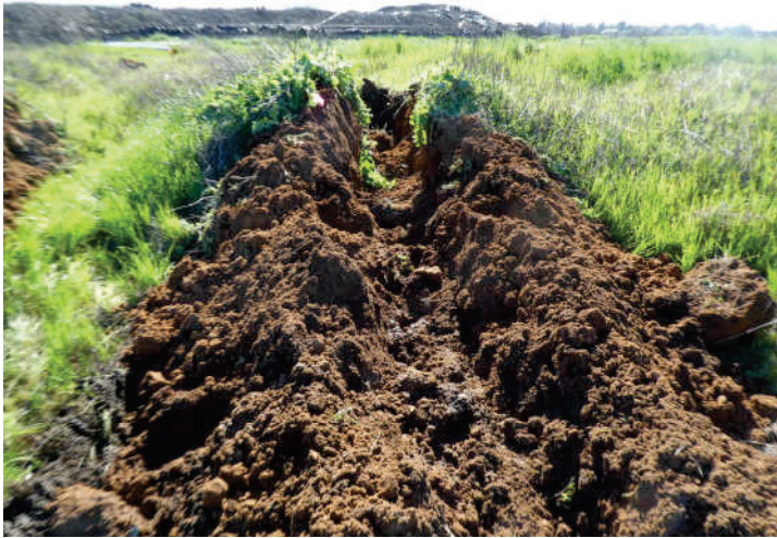
Photo #13: Northeastern soil piles Trench T-10
