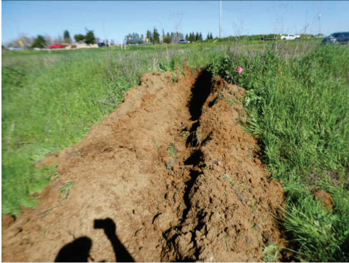
Photo #7: Northeastern soil piles Trench T-5
