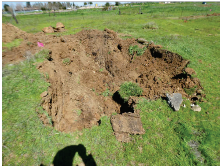
Photo #32: Western soil piles Trench T-9 - No significant staining or odor
