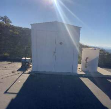
Photo 4: Looking East toward existing OSG unit.
