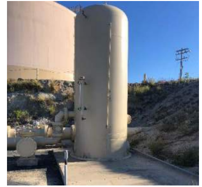
Photo 3: Looking North toward the existing surge tank.
