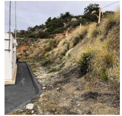
Photo 15: Looking West behind the existing electrical gears.
