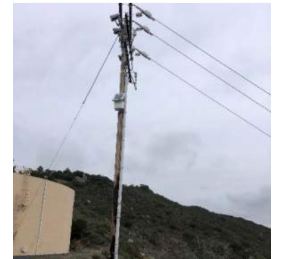
Photo 21: Looking North at the existing telecommunications pole onsite.
