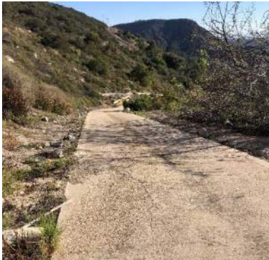
Photo 7: Looking Northeast at the main driveway.
