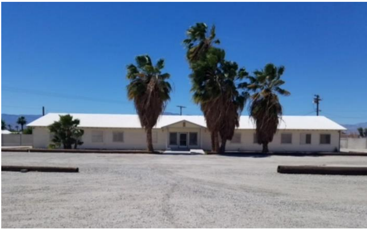
Photo 3: View west from Grapefruit Blvd. towards J26 Date Growers Building (i.e., “white house”) to be demolished.
