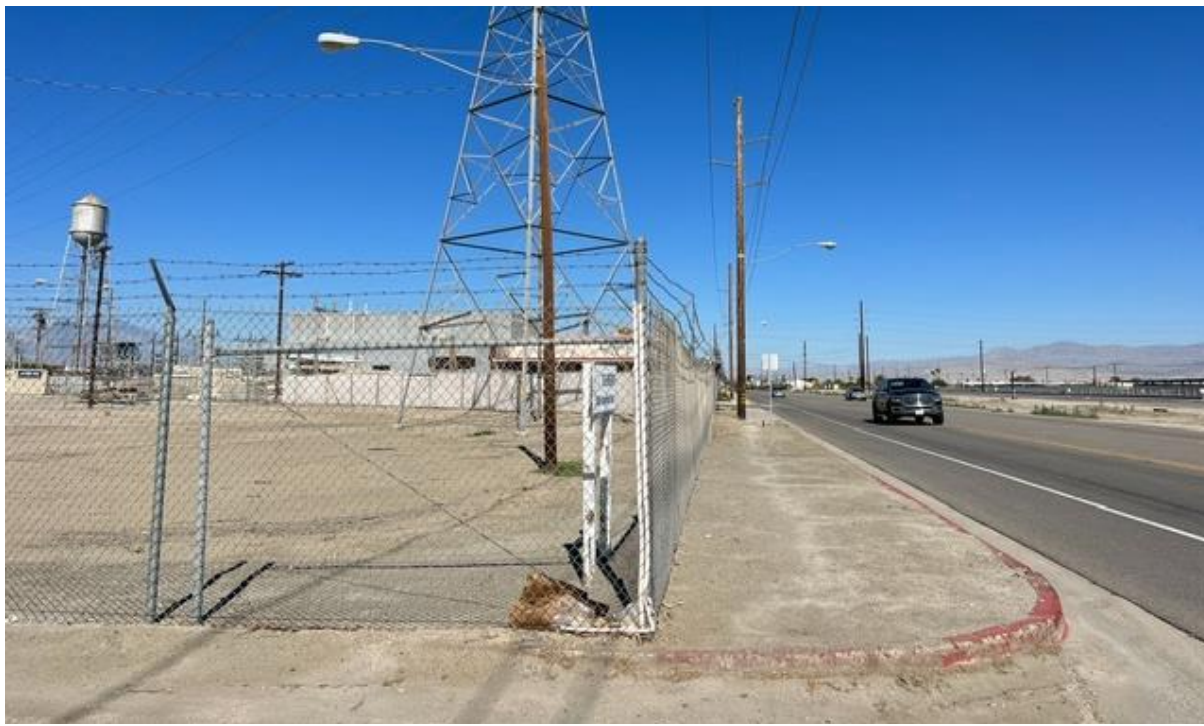
Photo 1: View north along Grapefruit Blvd. from entrance to Grapefruit Switching Station towards existing poles.
