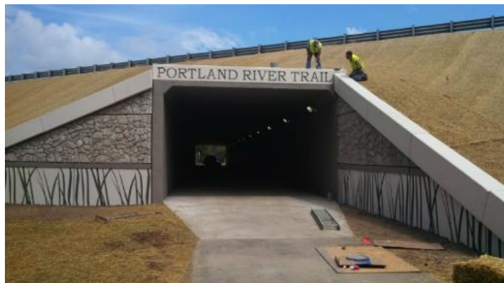
Figure 3: Example Trail Box Culvert Crossing
