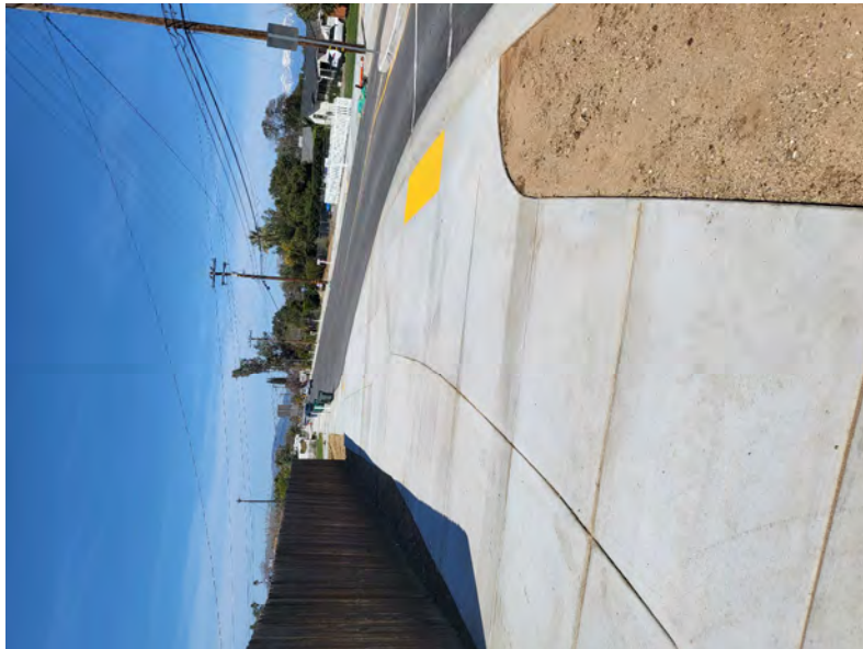
Photograph 3 - Looking W. down County Line Road (pipe installation)
