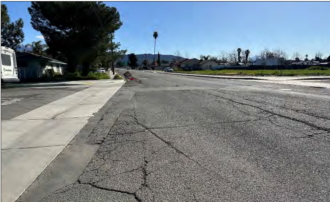
Figure 5-2 The northwest corner of 4th Street and County Line Road, facing southeast.
