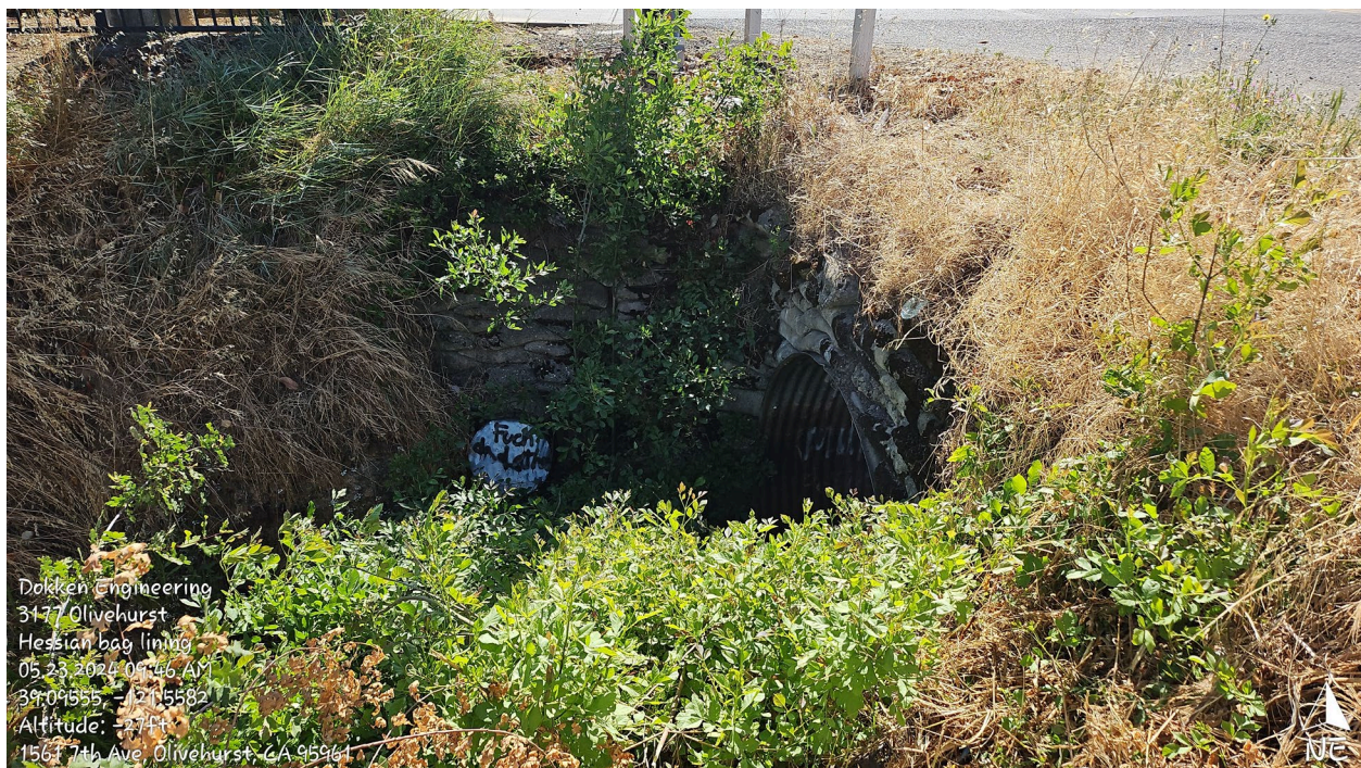
Photo 8. View of stacked Hessian Bags used as lining for the culvert under 7 th Avenue. View facing east/northeast.
