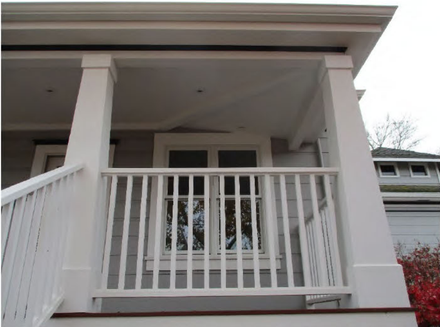
Photo showing a pair of vinyl windows, set inside an enlarged window opening.
