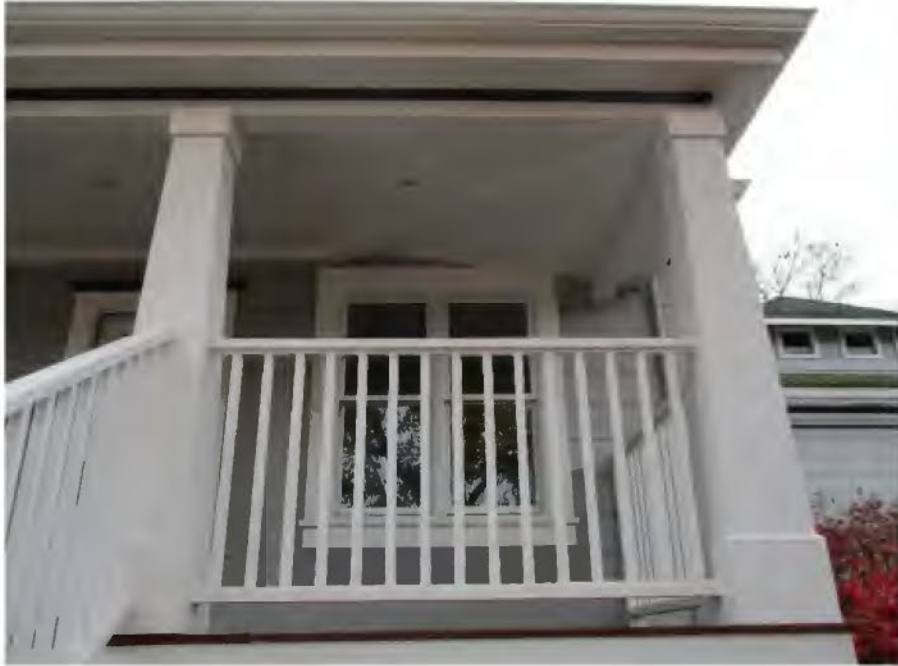
Figure 20. Photo showing a pair of vinyl windows, set inside an enlarged window opening.
