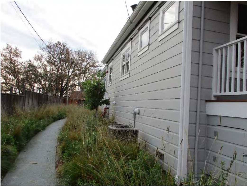
Figure 22. Photo showing the east elevation, facing south.
