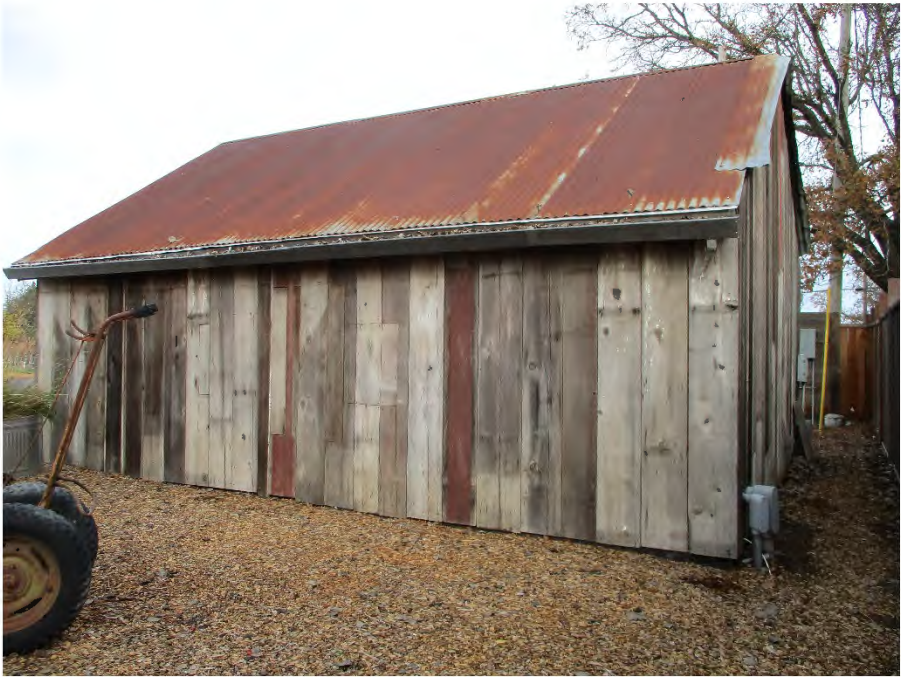
Photo showing north elevation, facing south.
