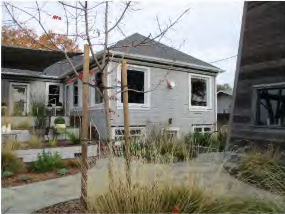
Figure 24. Photo showing the south elevation, facing north/northeast.
