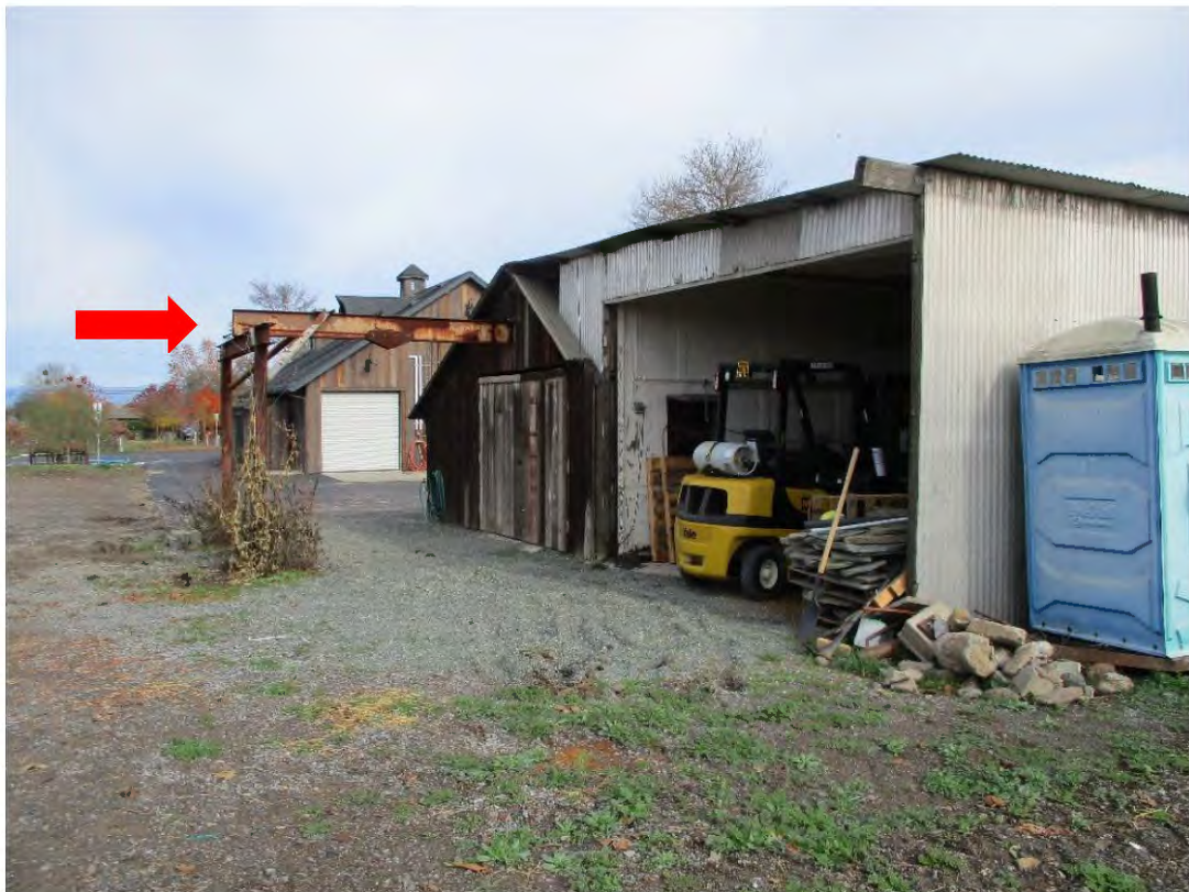
Figure 34. Photo showing overhead steel hoist, facing north.
