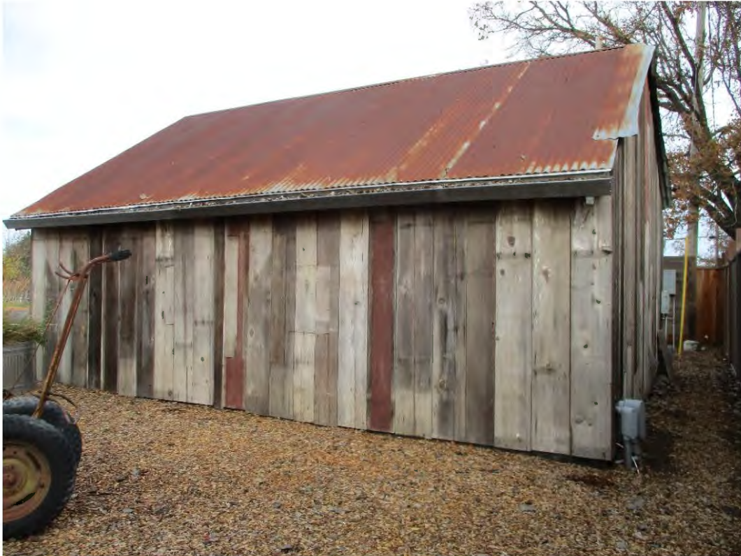
Figure 30. Photo showing north elevation, facing south.
