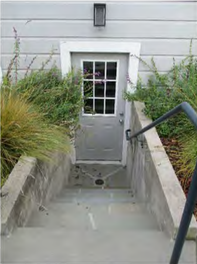
Photo showing the rear basement entry stairs and door.
