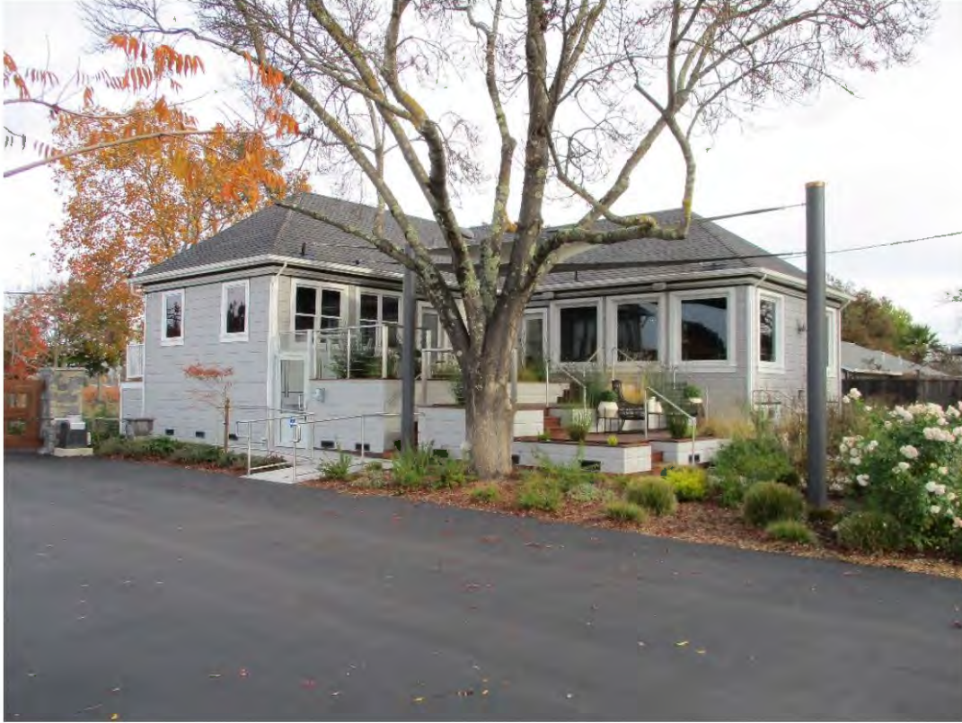
Figure 26. Photo showing the west elevation, facing north/northeast.
