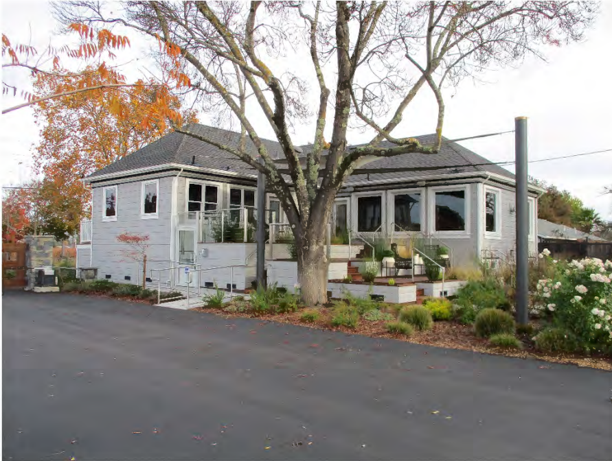
Photo showing the west elevation, facing north/northeast.
