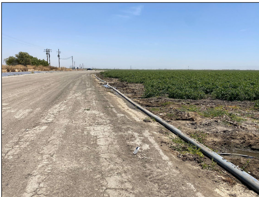
Figure 7. Overview of well 2, looking south.
