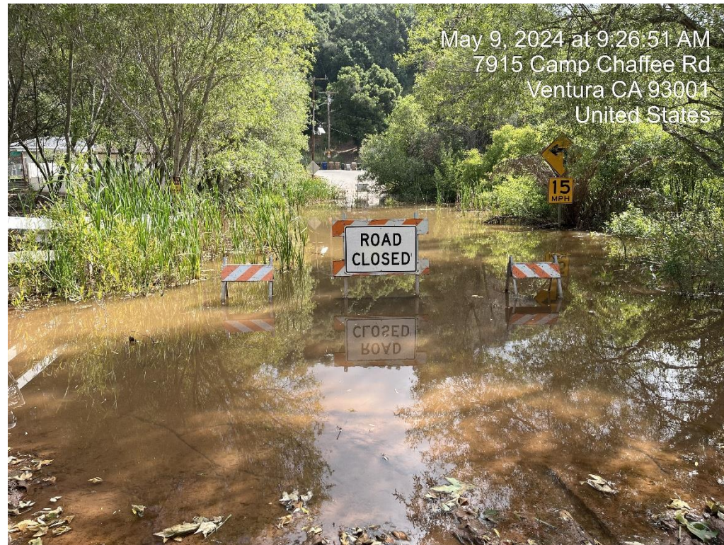
Image 1. Flooding at Camp Chaffee Road crossing taken 5/9/2024. This has been flooded and impassible since January 2023.
