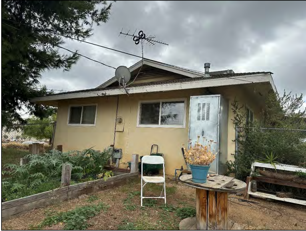
Image 10: View southeast of the north elevation.
