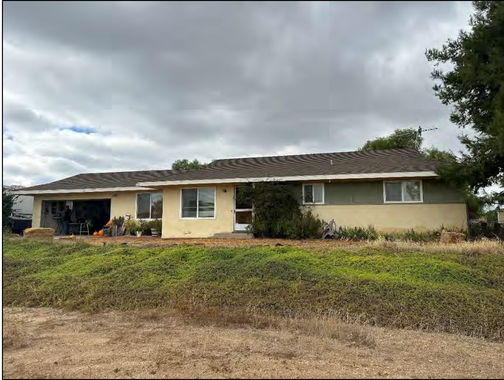
Image 2: View southwest of the east elevation.
