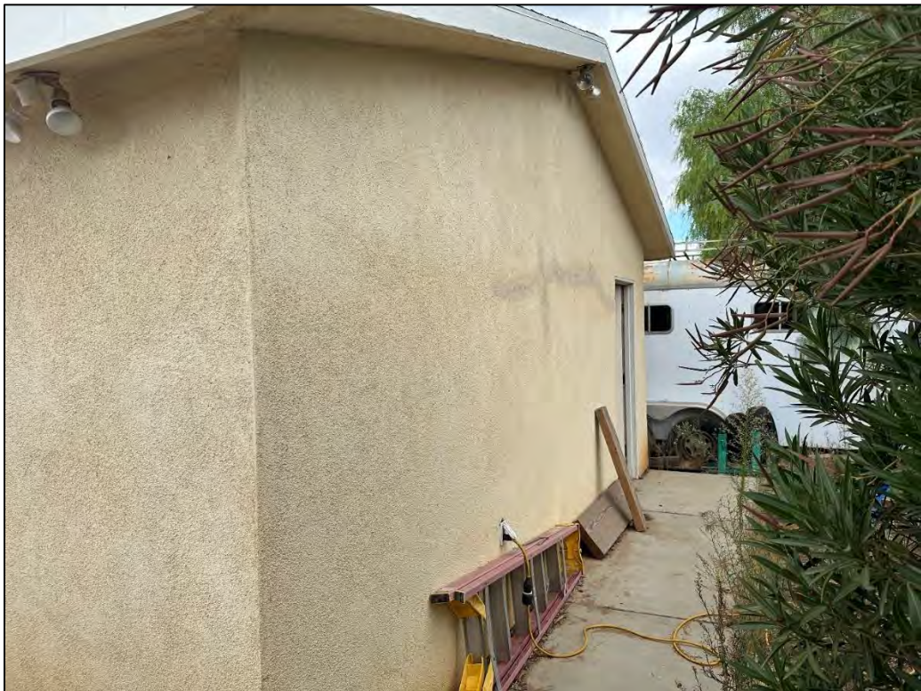
Image 13: View west of the north elevation of the garage.
