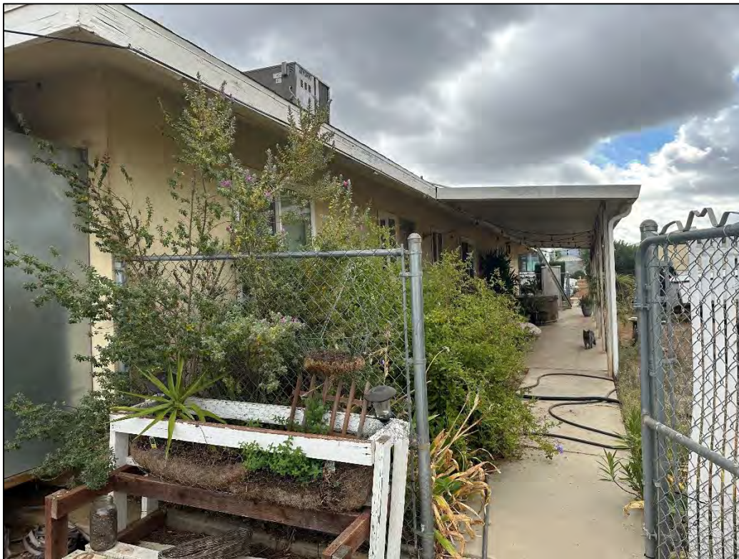
Image 11: View south of the covered walkway at the west elevation.
