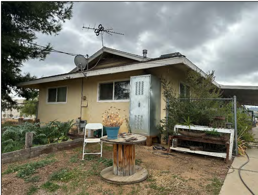
Image 9: View southeast of the north elevation.
