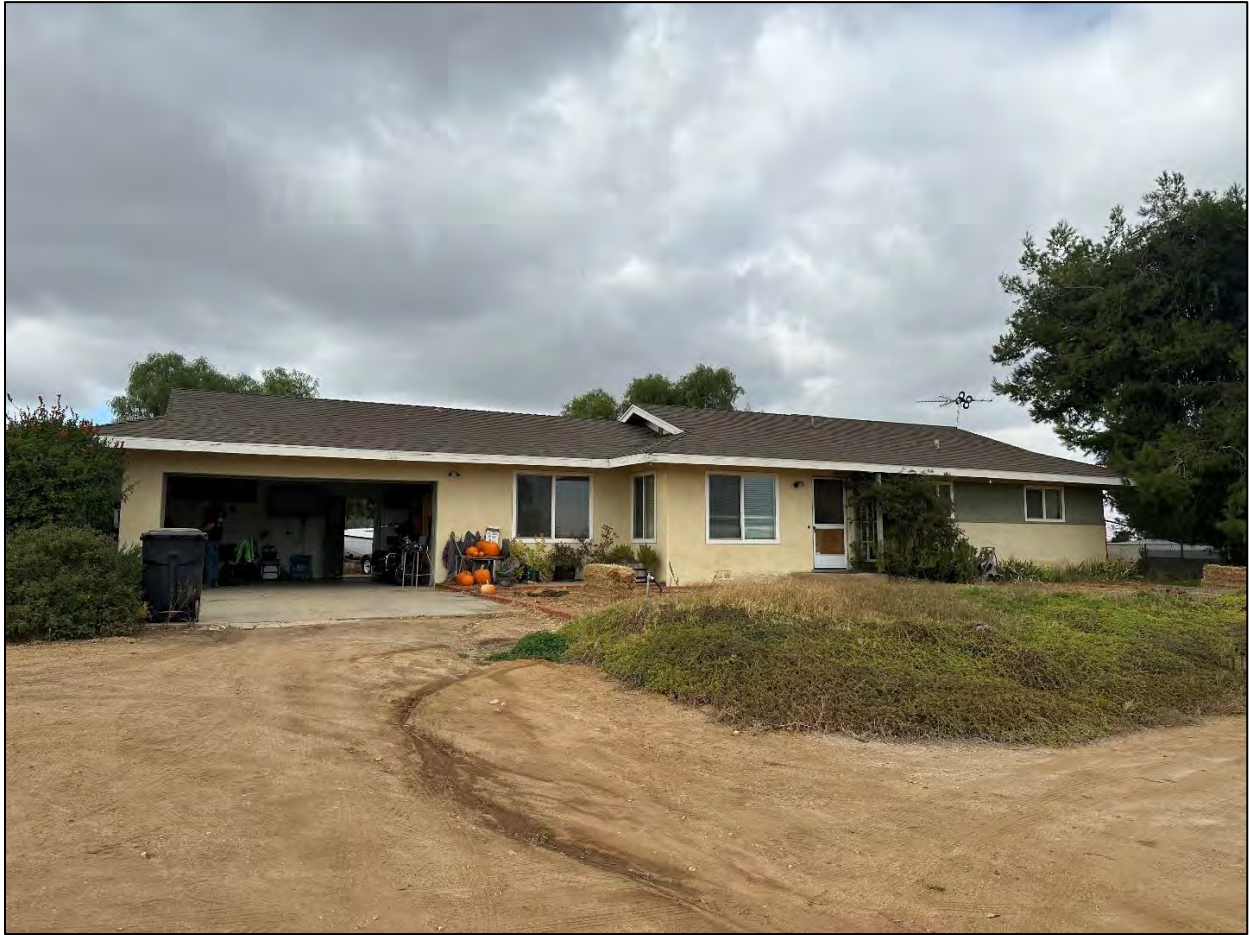
Image 1: View northwest of the front (east) elevation of the residence.
