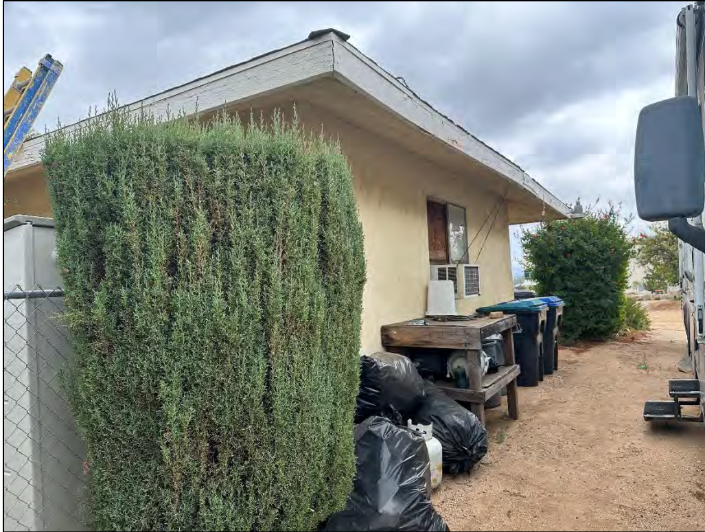
Image 6: View northeast of the south elevation.
