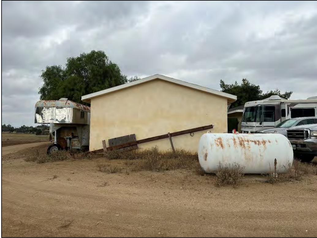
Image 14: View north of the south elevation of the garage.
