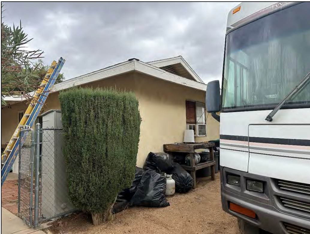
Image 5: View northeast of the south elevation.
