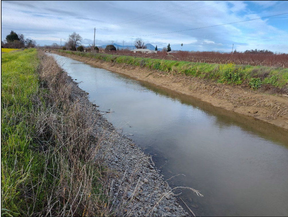
Photograph 1. Sutter-Butte Main Canal looking southwest.
