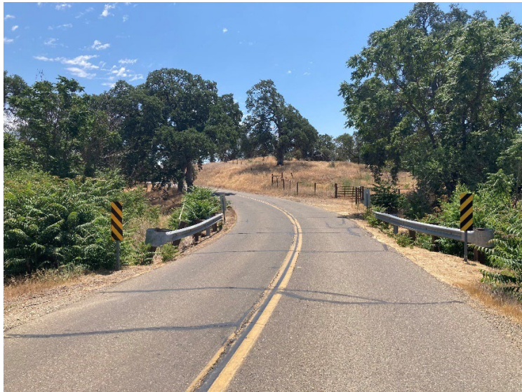
Overview of the Project area from School House Road. Taken facing southeast.
