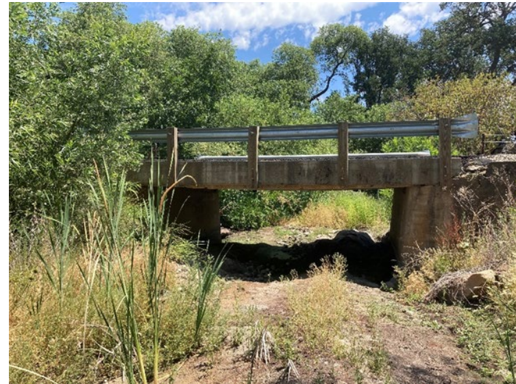
Overview of current School House Road Bridge from Owens Creek, taken facing east.
