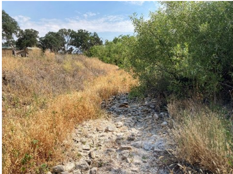
Owens Creek upstream of existing bridge. Taken facing northeast.
