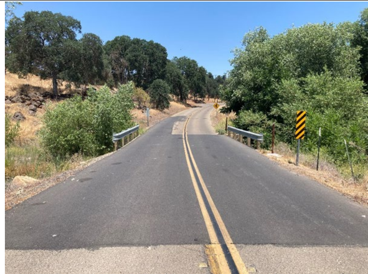
Overview of current School House Road Bridge, taken facing north.
