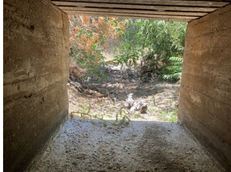
Ephemeral drainage and culvert under School House Road. Taken facing west (downstream).
