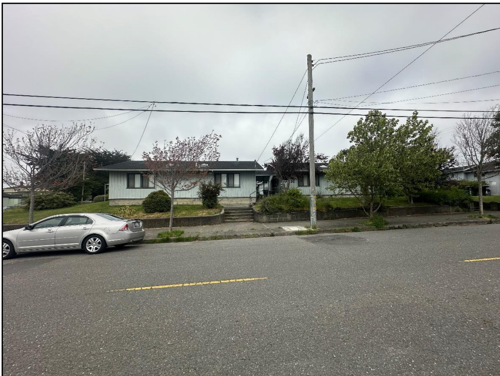
Photo 2: View of Project Site from C Street, view towards east
