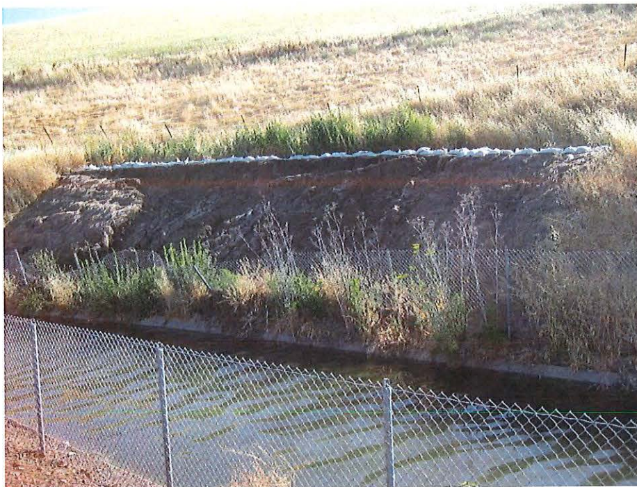
Photo 1. Example of Repairs from 2017 Storm Damage Repairs - Before
