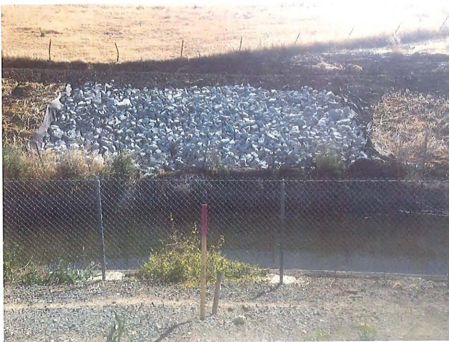
Photo 2. Example of Repairs from 2017 Storm Damage Repairs - After
