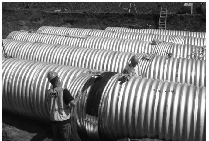
Tightening bolts on a corrugated band.
