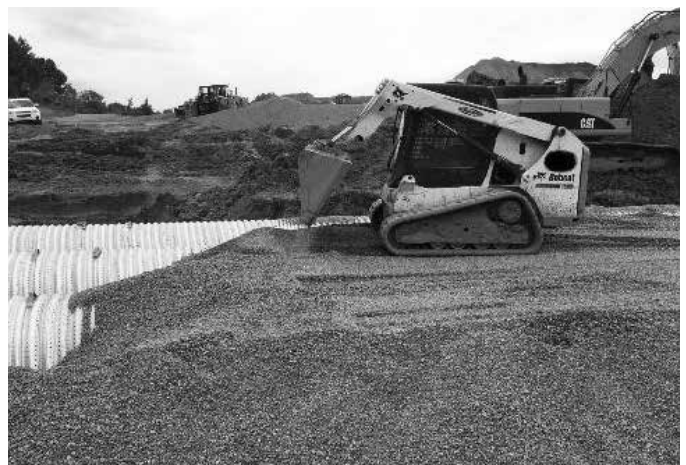
Examples of light, tracked, construction equipment used to place final cover over the pipe system.
