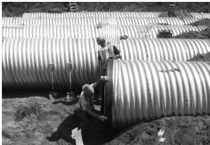
Installation of band with flat neoprene gasket.
