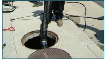
Cleaned easily with vac truck, without catch basin entry, and about 15 minutes is required for service.
