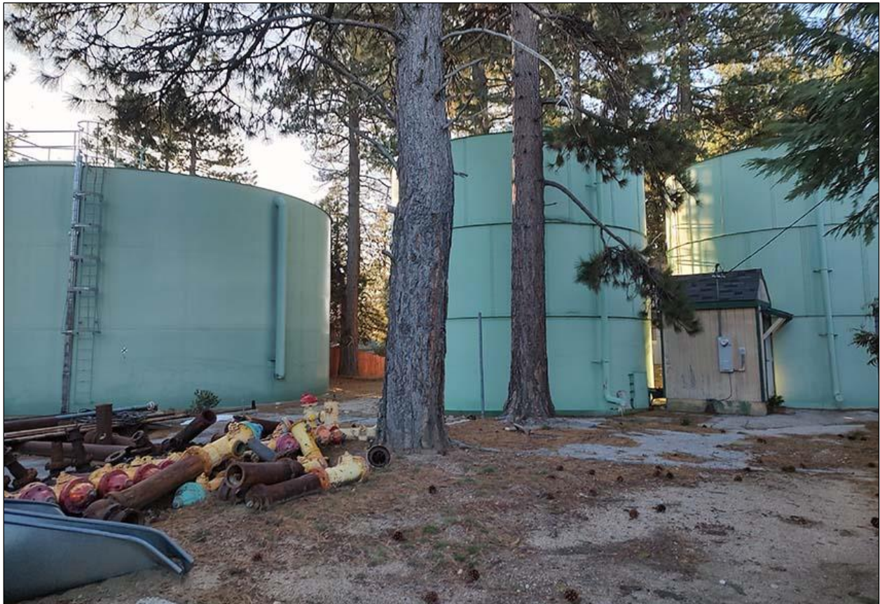
Figure 8. Reservoir tanks at 4103-1H. (Photograph taken on March 14, 2024; view to the south)
