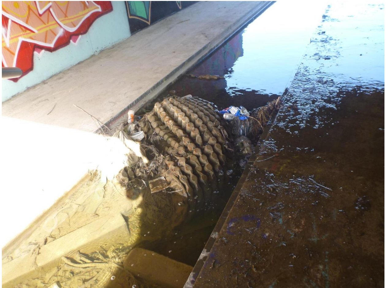
FIGURE 16: EXAMPLE PORTION OF CLOGGED WASHINGTON BAFFLES.
