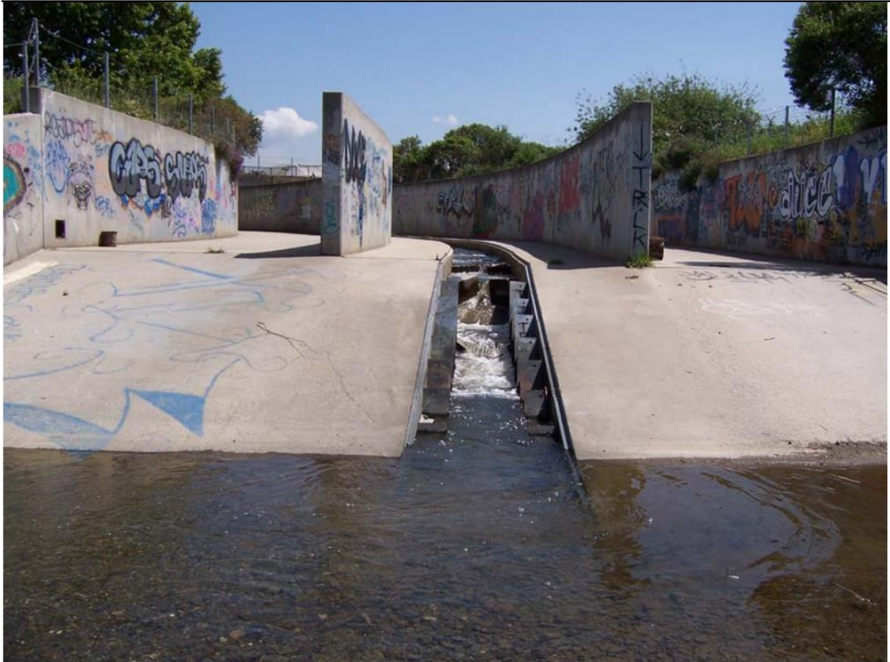
FIGURE 14: EXISTING DENIL FISH LADDER, CLEARED OF SEDIMENT, LOOKING UPSTREAM FROM SEDIMENT BASIN. PHOTO FROM EBRPD IN 2007.
