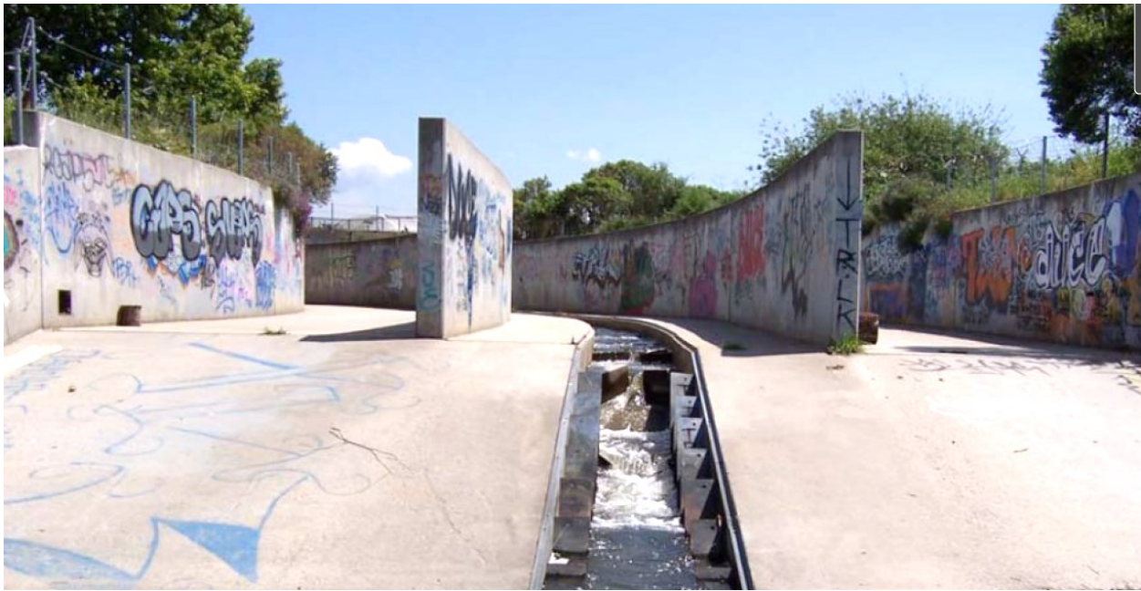
FIGURE 1 - 3: FISH PASSAGE STRUCTURE
