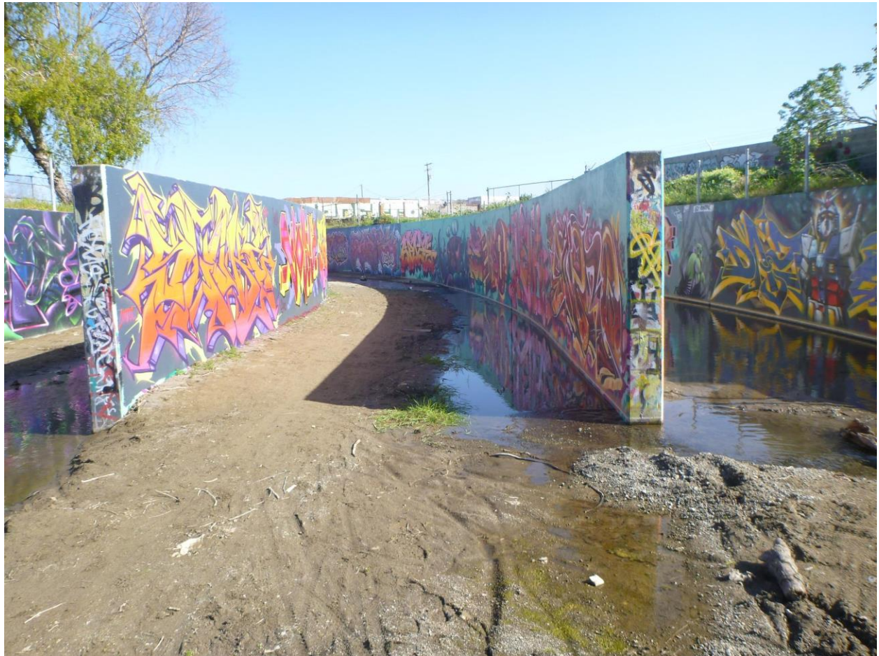
FIGURE 15: DENIL FISH LADDER, FILLED WITH SEDIMENT, LOOKING UPSTREAM FROM SEDIMENT BASIN. PHOTO FROM 2022.
