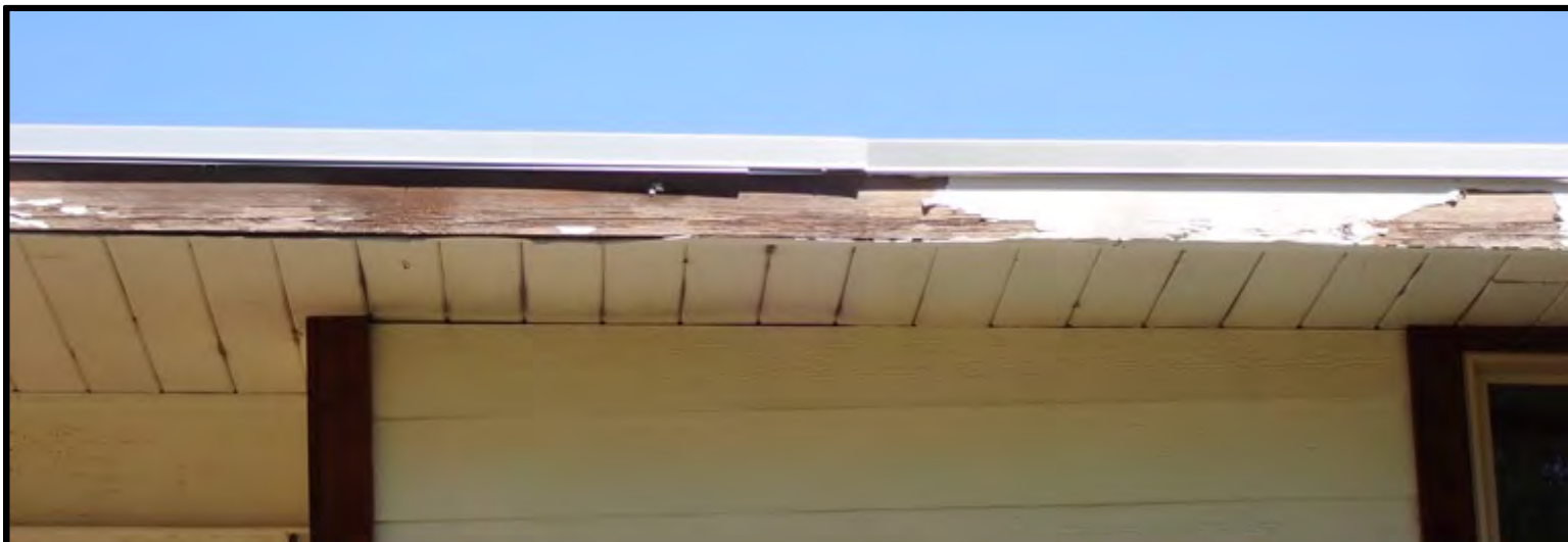
Image 4. View of the chipping paint on the western overhang of the mobile home located on the Southern end of the Subject Property.
