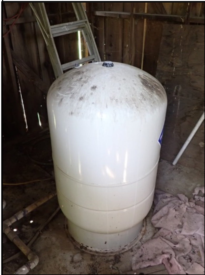
Image 5. View of the aboveground water pressurization tank inside the well house.
