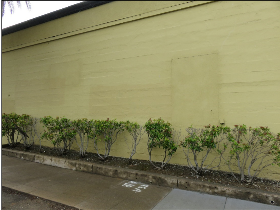
Detail of infilled openings in the exterior concrete wall, north façade of 11 South B Street
