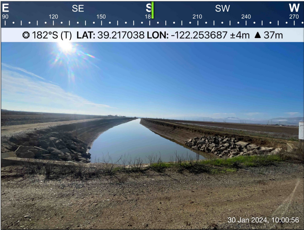
Photograph 16 Overview of the Glenn-Colusa Canal south of the siphon.
