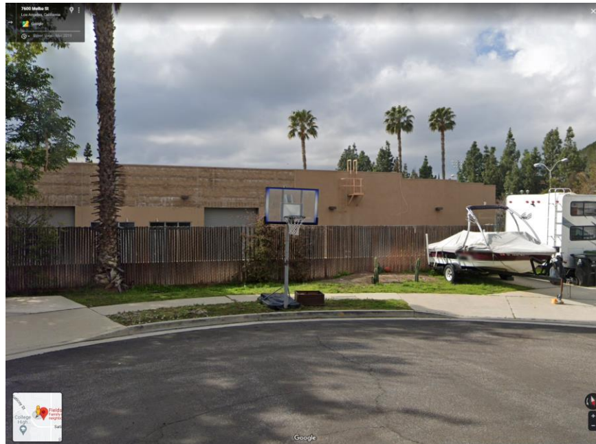
Figure 3: Google street view showing the full-cutoff wall-mounted lighting on the north side of the existing commercial building at the eastern end
